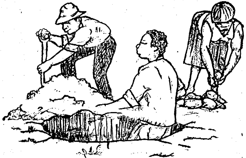
DIGGING A WATERWELL
