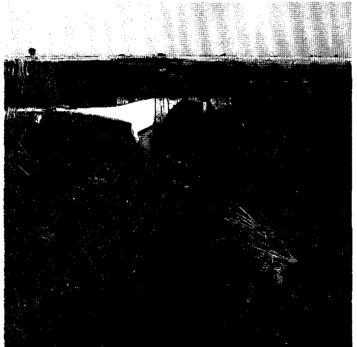
Photo 18 Modern drainage ditch for seepage flow with sluices to regulate water levels for irrigated rice cultivation. Such stagnant water bodies may create health hazards. Namushakonde.
