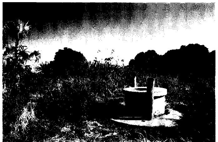
Photo 37 Shallow well lined with concrete at floodplain edge in Mongu; note that the winch has been removed.
