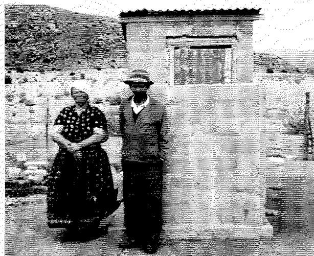
Ventilated improved pit (VIP) toilet in Nourivier, Namaqualand
