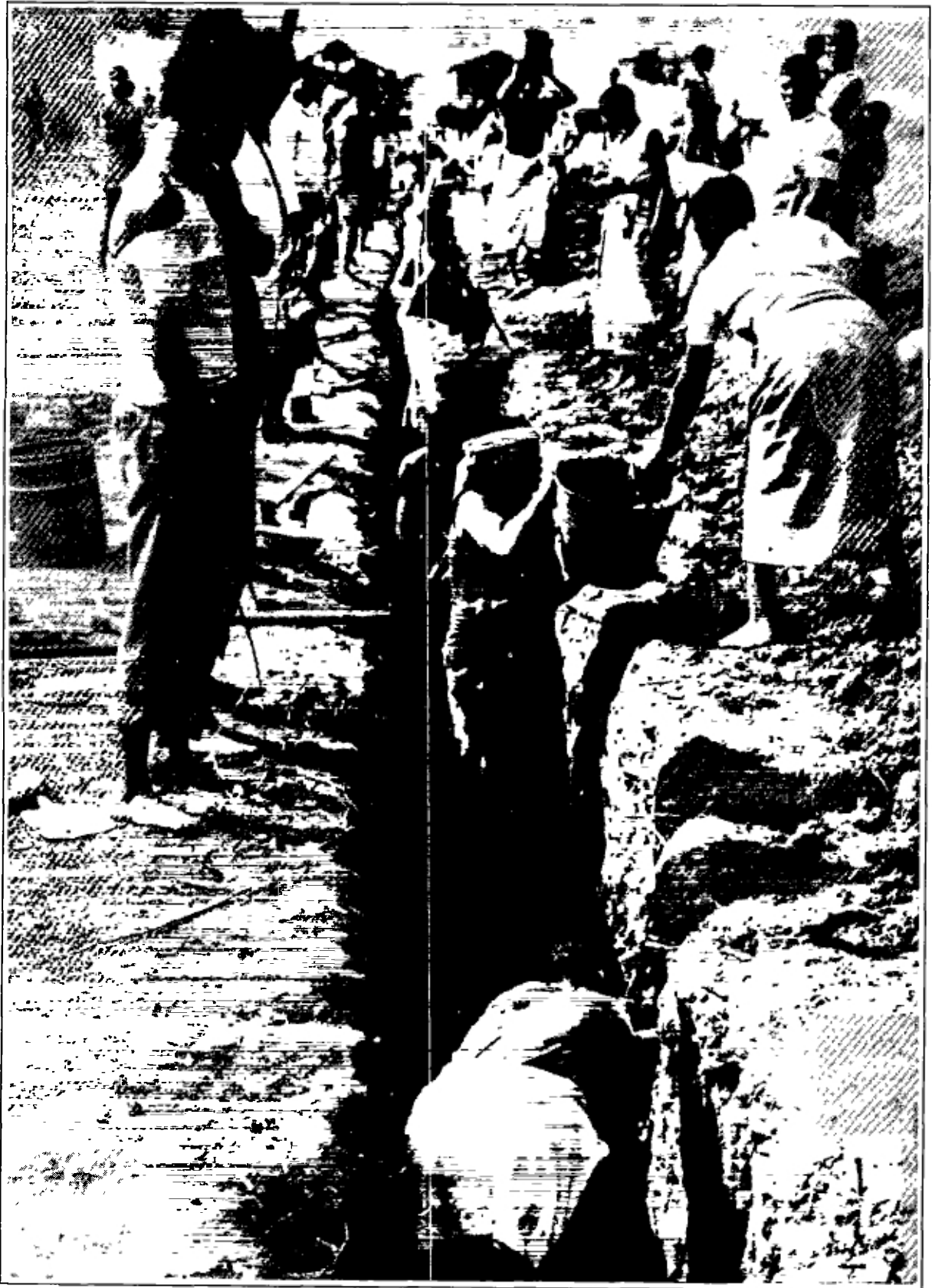
Figure 13. User participation in trench digging
