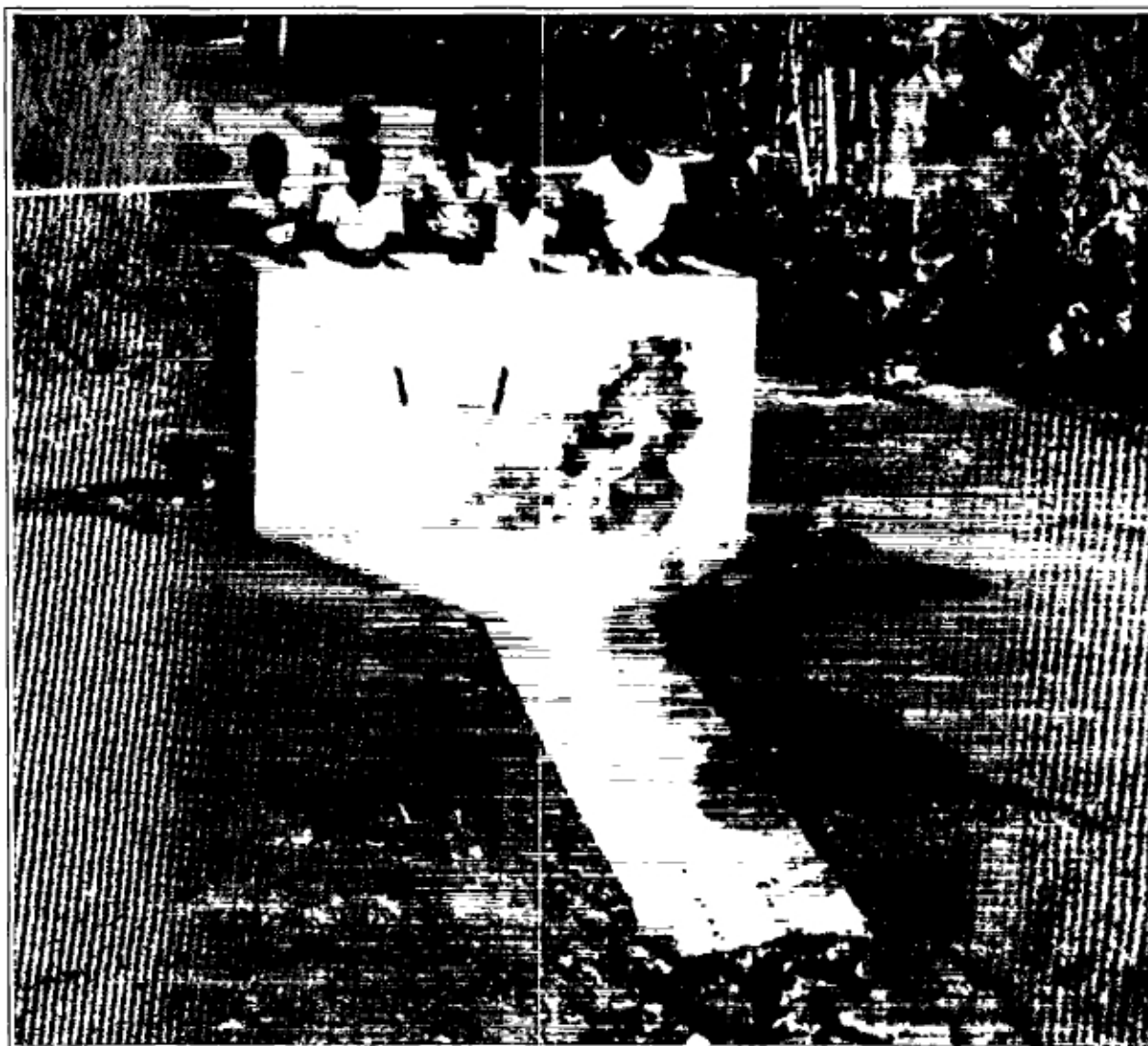
Figure 15 Users at clothes washing slab, drain and soakaway
