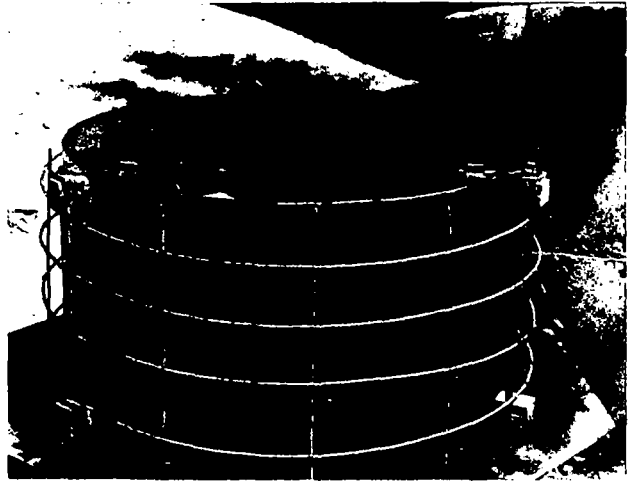
50 cm BUSE MOLD showing triangle and re-rod placement
