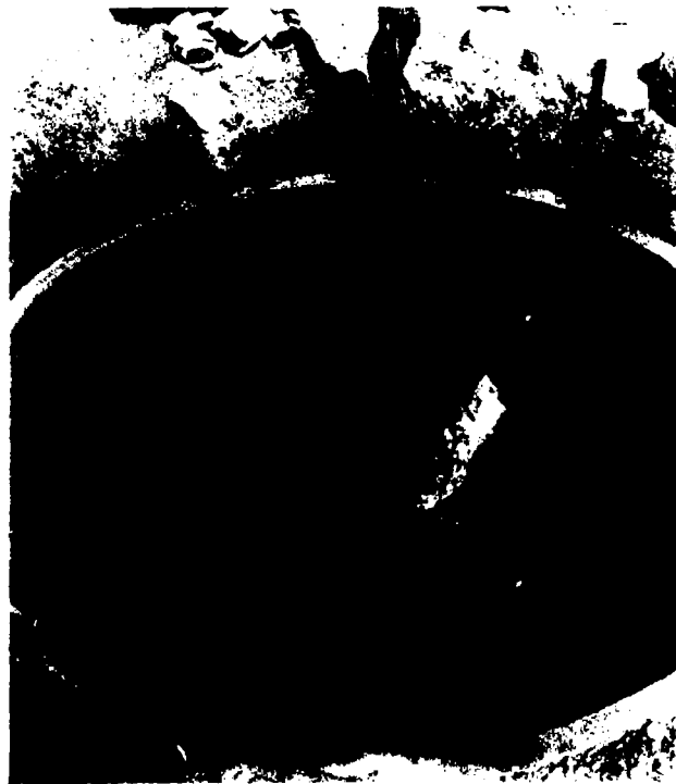
COMPLETE CASTING which has been watered. The small holes allow water flow into the well
