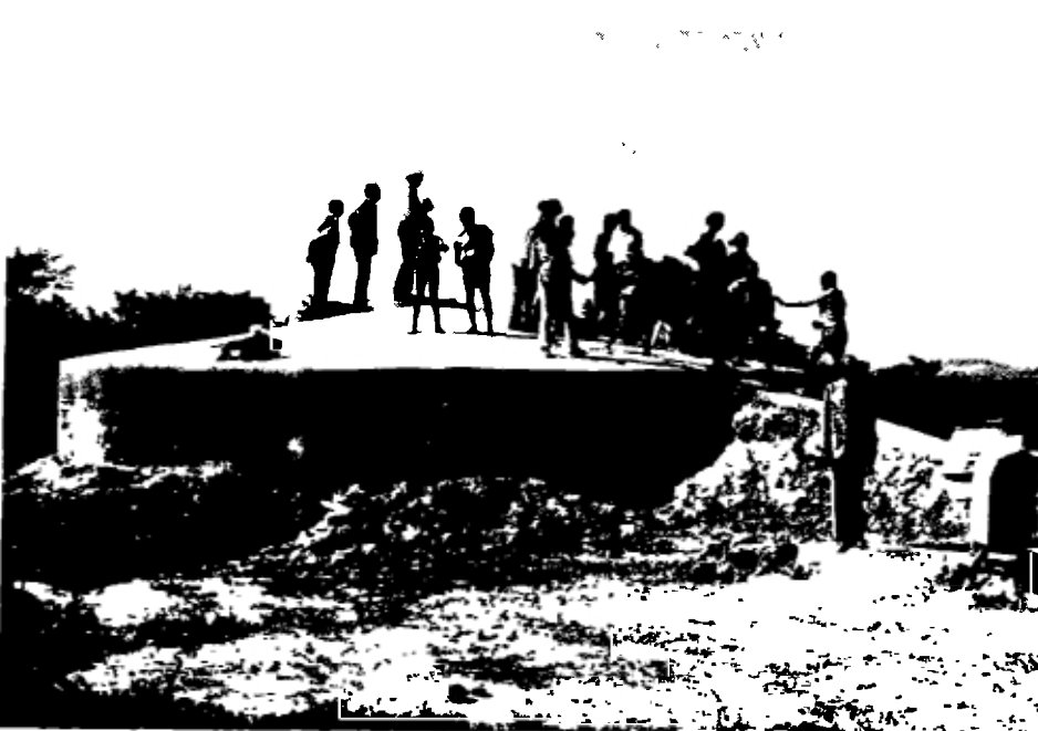
Photo 6. 30,000 gallon storage tank, Champira South.
