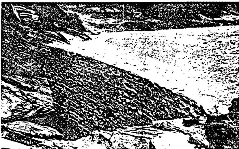
Sand dam in South-West Africa built of rock and mortar. (O. Wipplinger)
