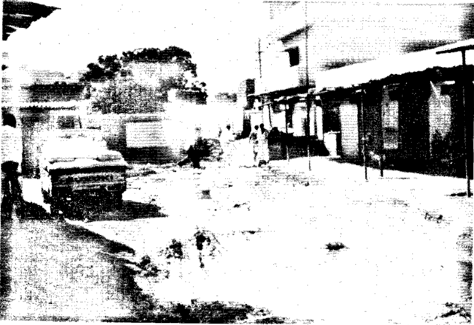
Condition of road before external sewerage development in Mujahid Colony
