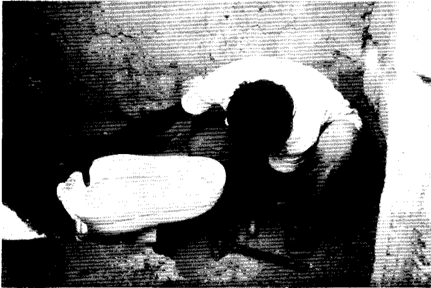
Figure 3.8 Mason installing a pan
