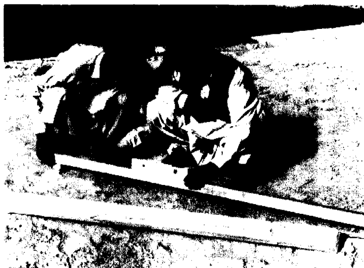
THE PRECISE SLOPE IS ESSENTIAL FOR WATERPROOFING
