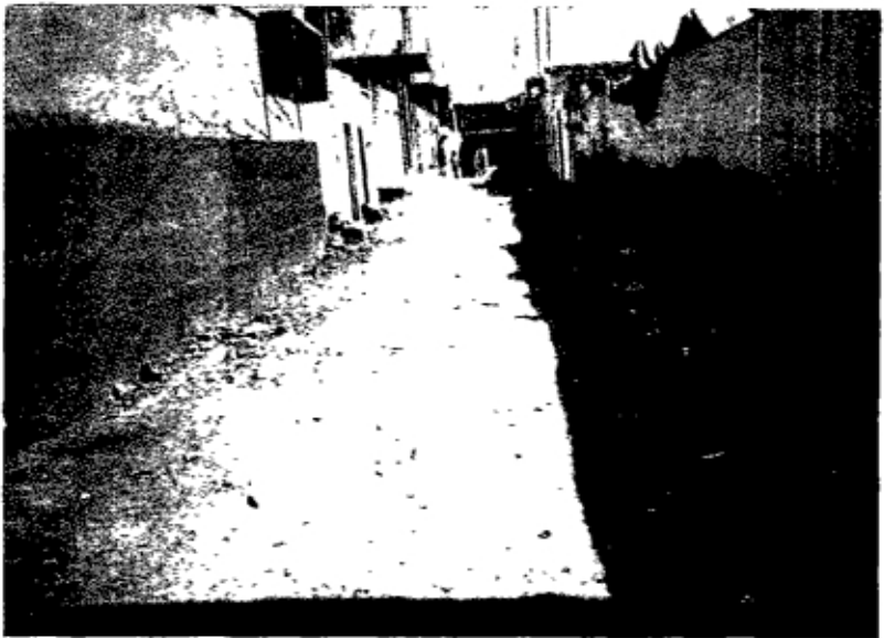
Manzoor Colony Karachi: a lane after the completion of sewer line
