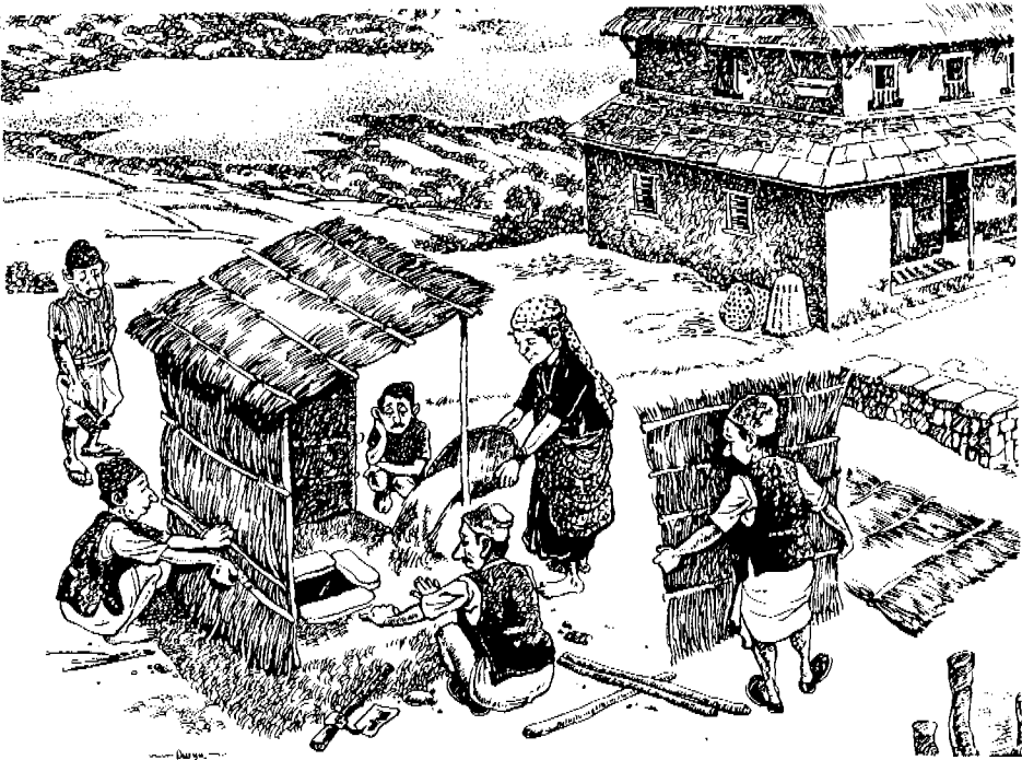
Construction of a latrine using locally available materials; picture taken from health education flipchart
