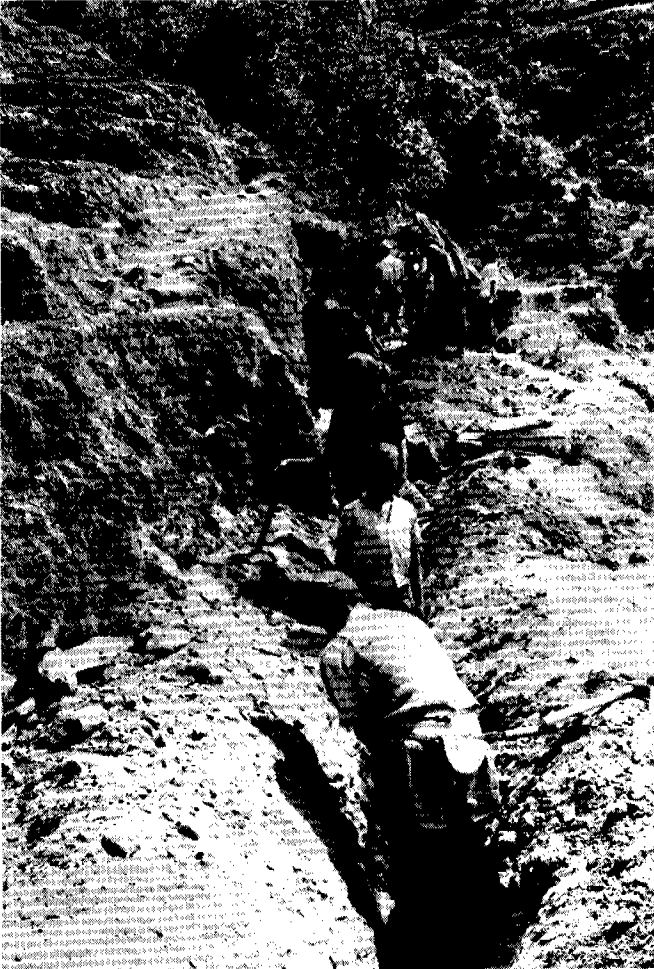
Trench digging by voluntary community labour
