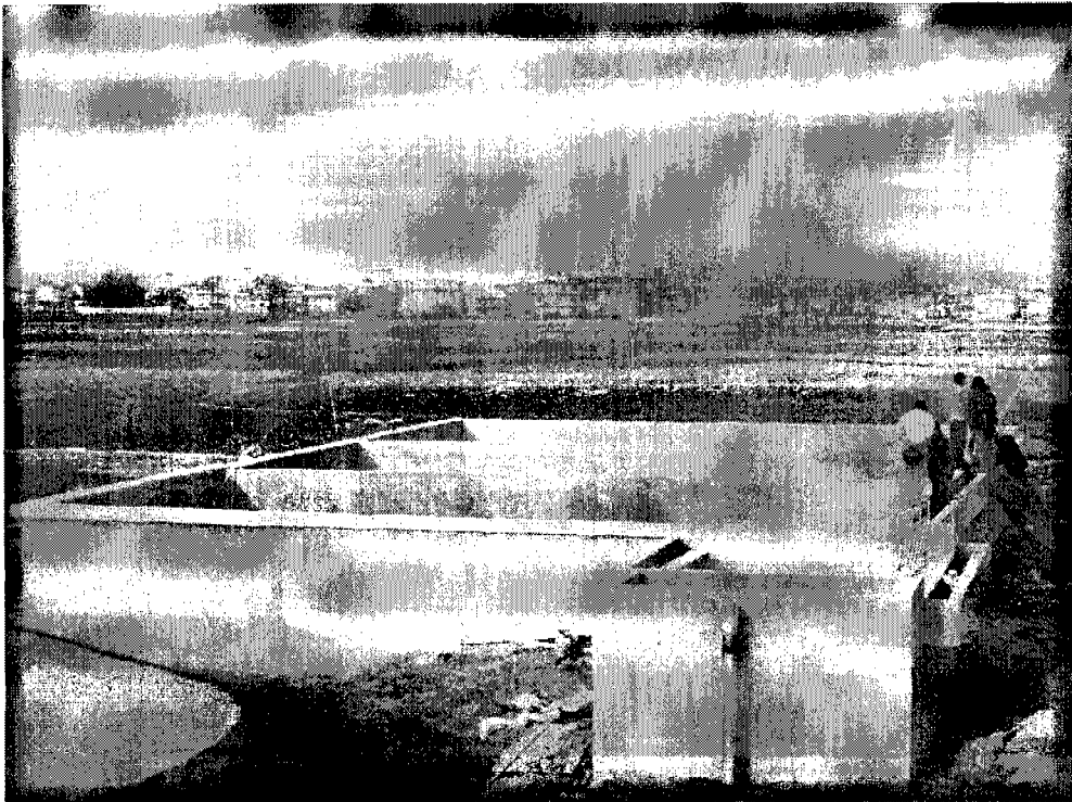
Picture 4: Completed civil structure of the Slow Sand Filter
