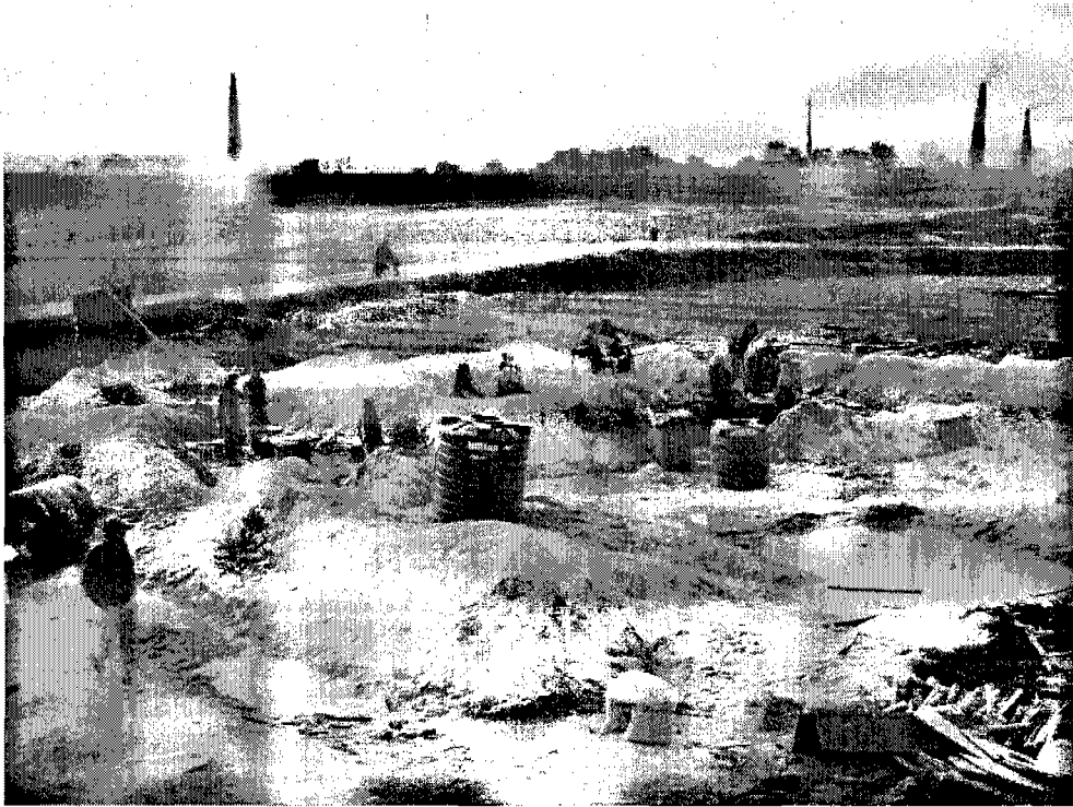
Picture 7. Preparation of filter media for Slow Sand Filter
