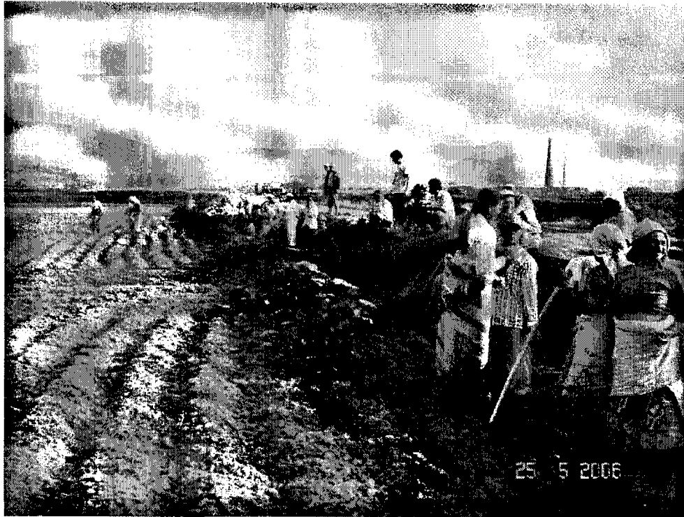
Picture 11: Community helping in laying of pipes for the water supply
