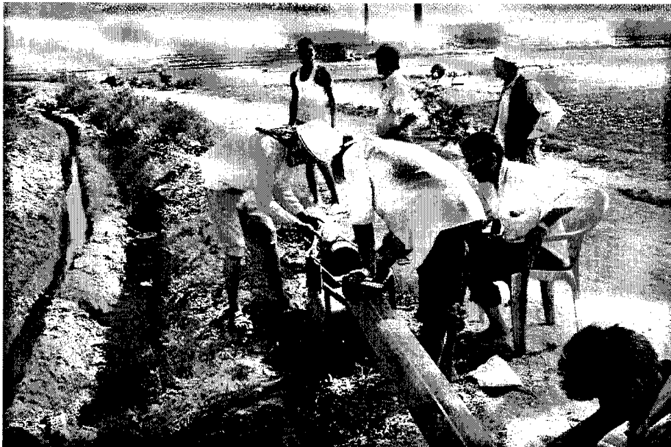
Picture 12: Plumber laying down pipe lines
