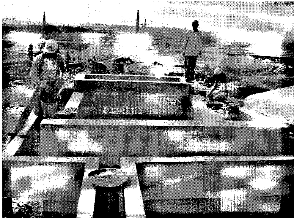
Picture 10. Civil structure of Tube Settler after completion
