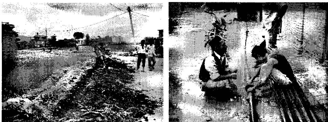
Picture 1: Water distribution work in Siddhipur
