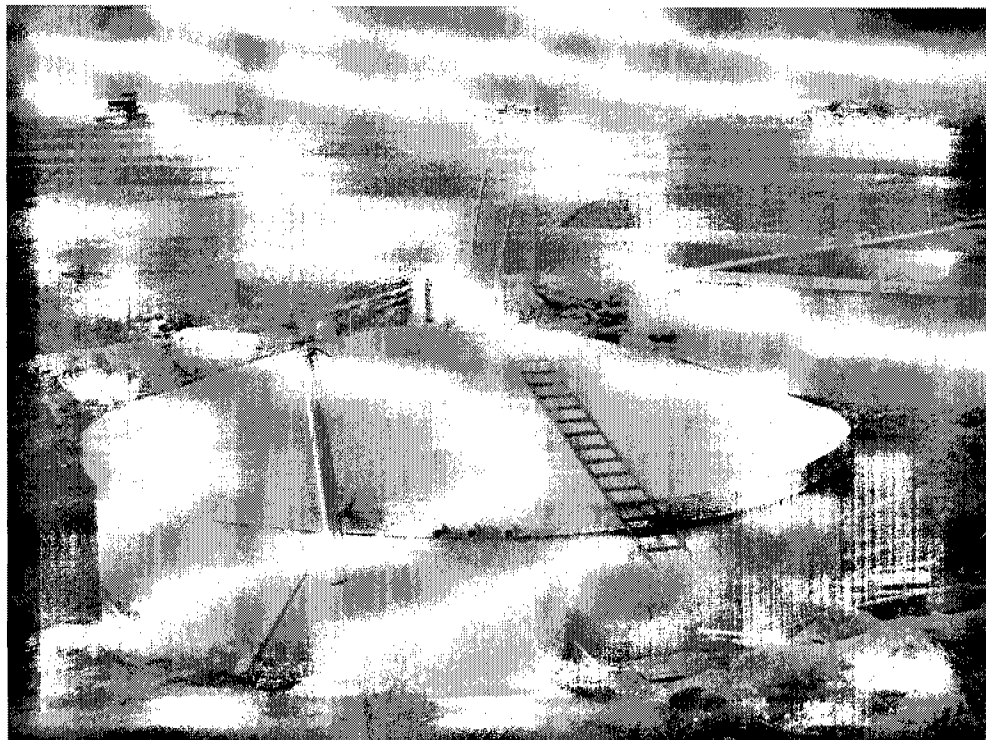
Picture 6: Completed civil structure of Reservoir Tank
