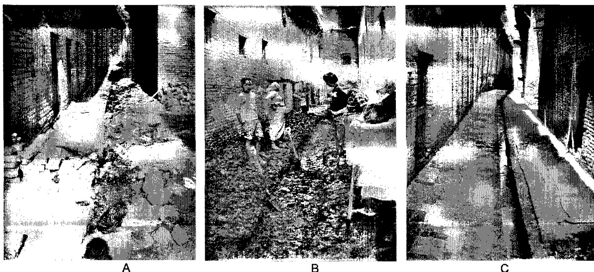
Picture 6: Pavement and Drainage work at Ramdhoka Galli
