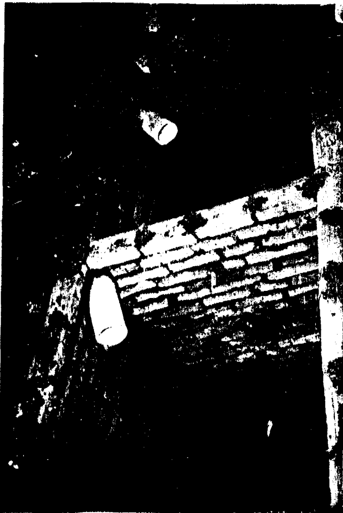
PHOTO 7 Pipes were used to simplify the drain construction. Kirtipur-Dec.1981
