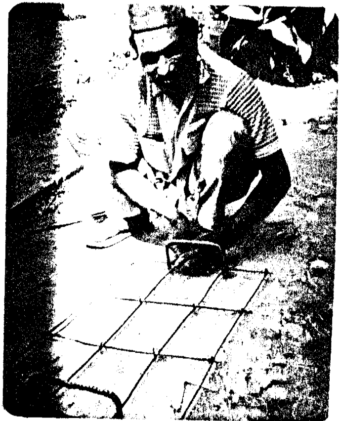
PHOTO 21 Local mason at Dhadhikot in being trained to make the reinforced cover Slabs Dhadhikot 1982
