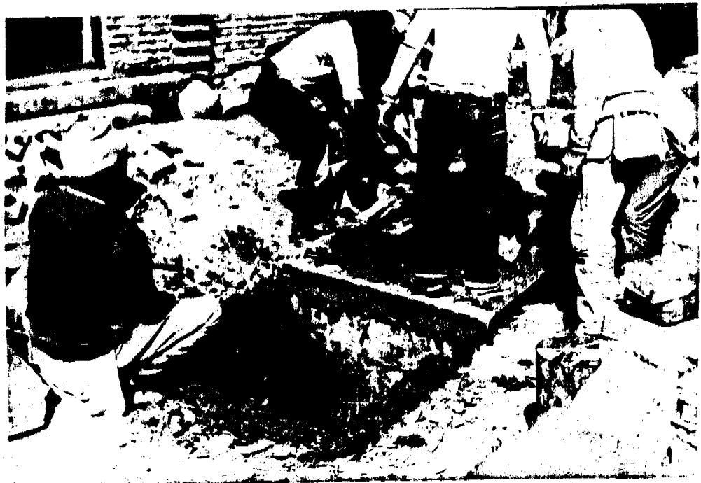
PHOTO 14 One of the pit is covered with Slab, A layer of mud is necessary to prevent leaking of foul gas from the pit. Thimi 1982
