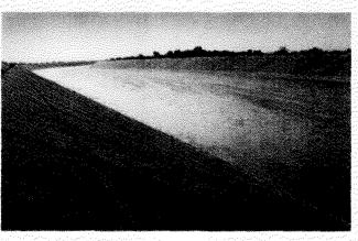
groove cutting. This would improve the rugocity co-efficient resulting in better flow condition.
