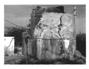
The earthquake also annihilated or damaged greatly the lifeline of the villages - the water-related infrastructure. The impact of the earthquake on piped water supply systems, in-village facilities, water harvesting systems, and traditional water storage structures meant that there was no drinking water for the people. Restoring drinking water supply systems became an integral part of rehabilitation and reconstruction efforts.
