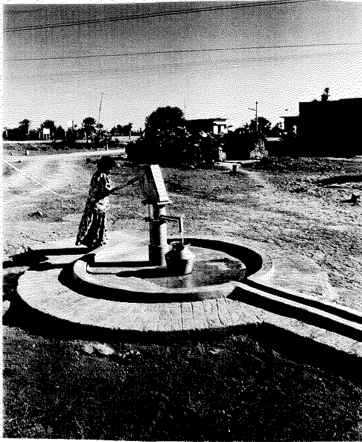
Photo 9 : Brick-lined platform constructed to ensure environmental protection of safe water source.
