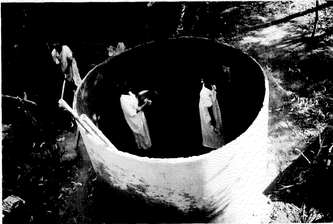
Photos 1 & 2 : Empowerment of women through mason's training for construction of rainwater harvesting structures.
