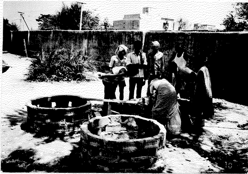
Photo 7 : A model of a twin-pit latrine being constructed for a sanitary park.
