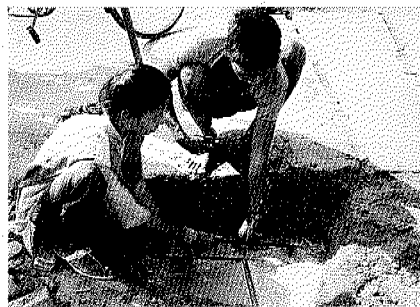
△ Disconnecting an illegal water connection
