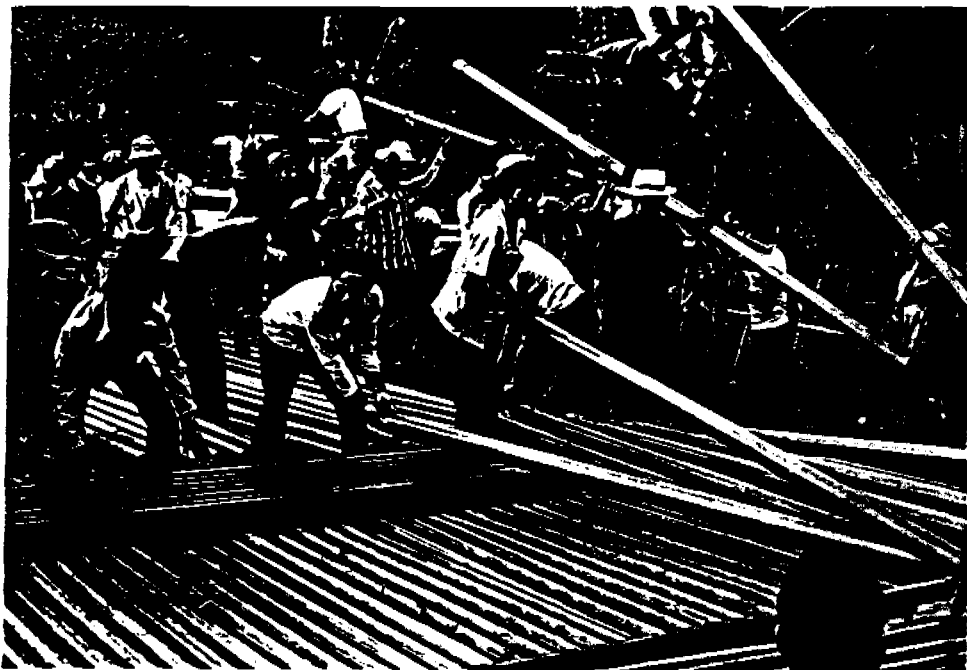
PVC pipes contributed by the Public Works' Water Supply Project for kampung Sukamulia
