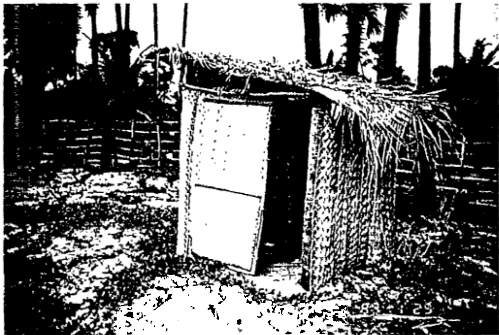
Simple but efficient latrine superstructure made from coconut leaves. The construction admits daylight and gives excellent cross-ventilation.
