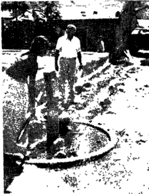
4. Bad Drainage and Platform
