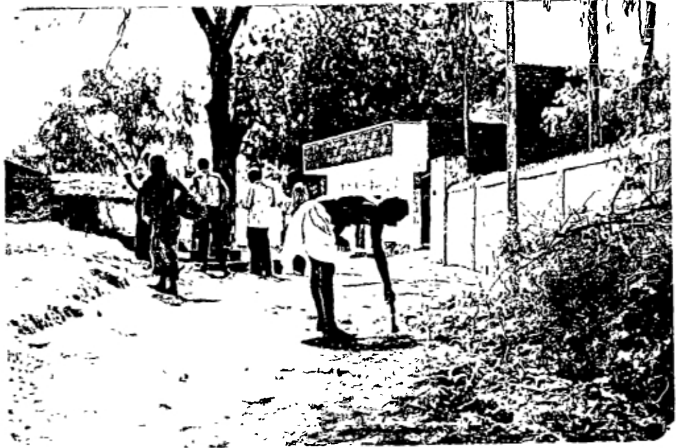
A: Cleaning a drain constructed with equal contribution by beneficiaries
