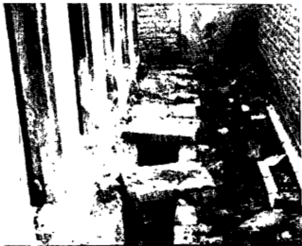
Faeces litter the entrance to the toilets; missing taps, damaged sewer connections and floors were typical.
