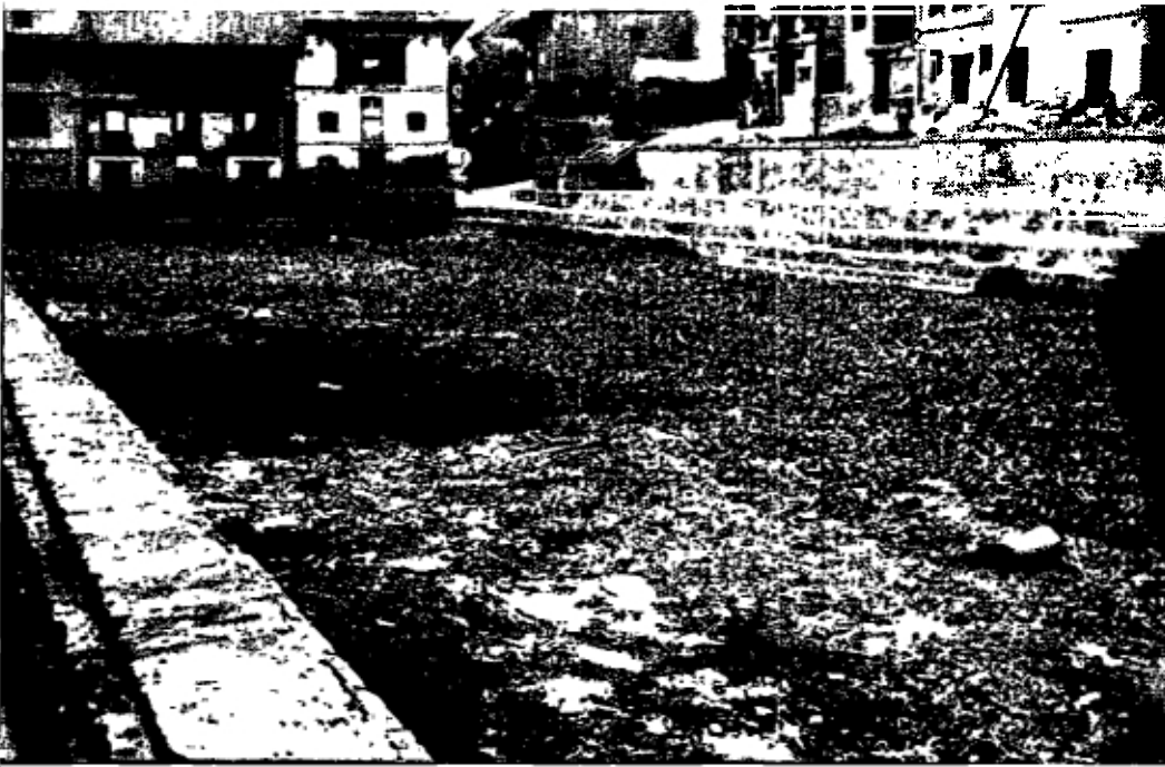
Renovated ponds again started to become dirty and polluted.
