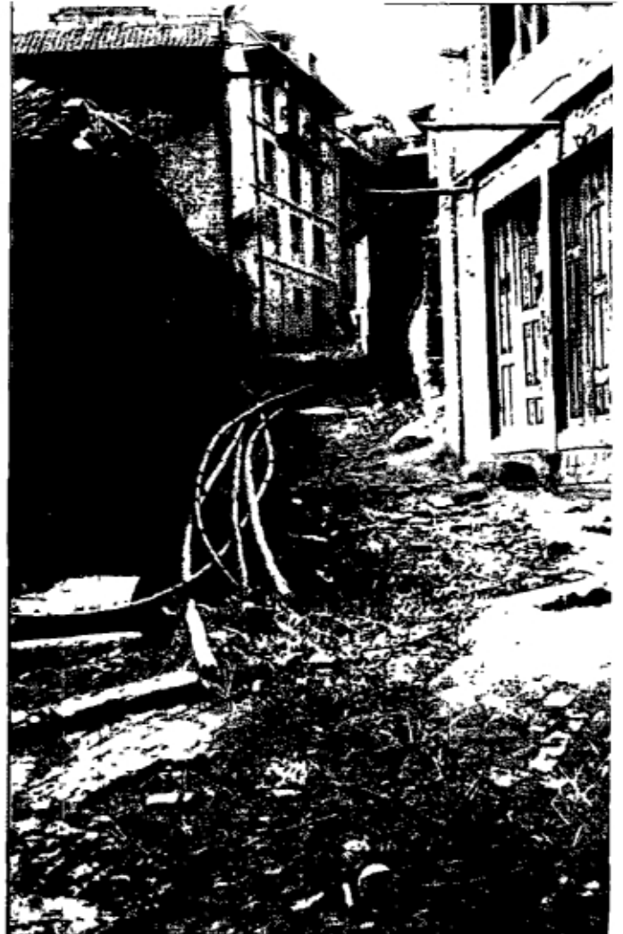
Unpaved streets worsened considerably.
