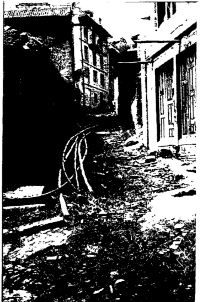
Unpaved streets worsened considerably.
