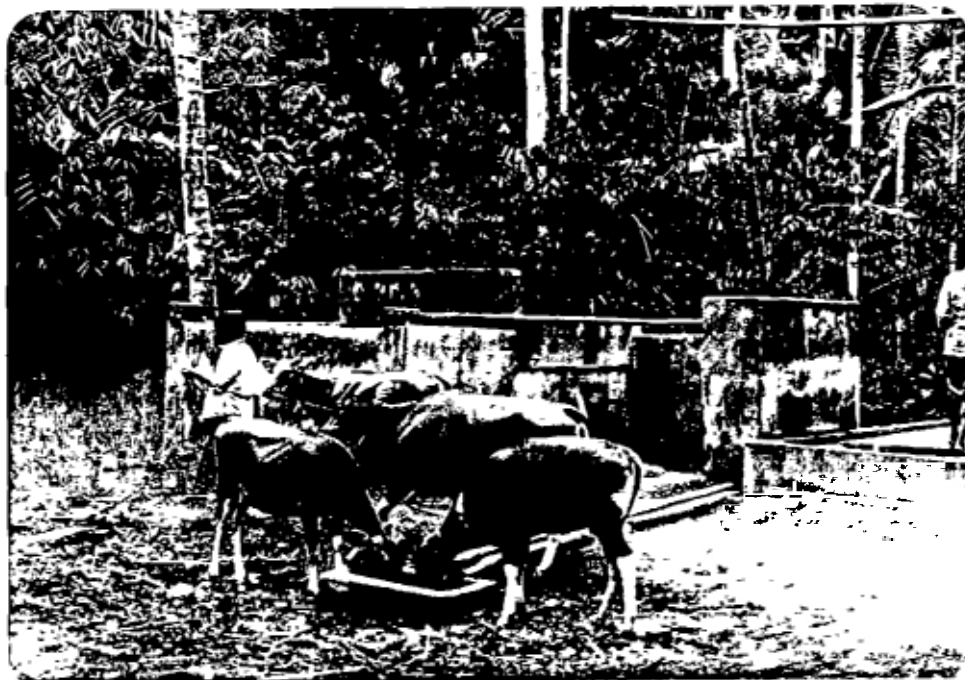
Hand dug deep well AID-type project in North Lombok. Approximately 100 families and their livestock use these sources. (Bathouses in the background behind cattle; well 30 meters deep with concrete rings)
