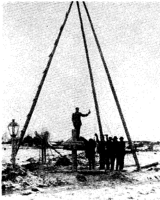
Fig. 6. Tube well construction in Mustasaari-Island close to Oulu in the 1930's (Northwestern Finland). (Photo: National Board of Antiquities).
