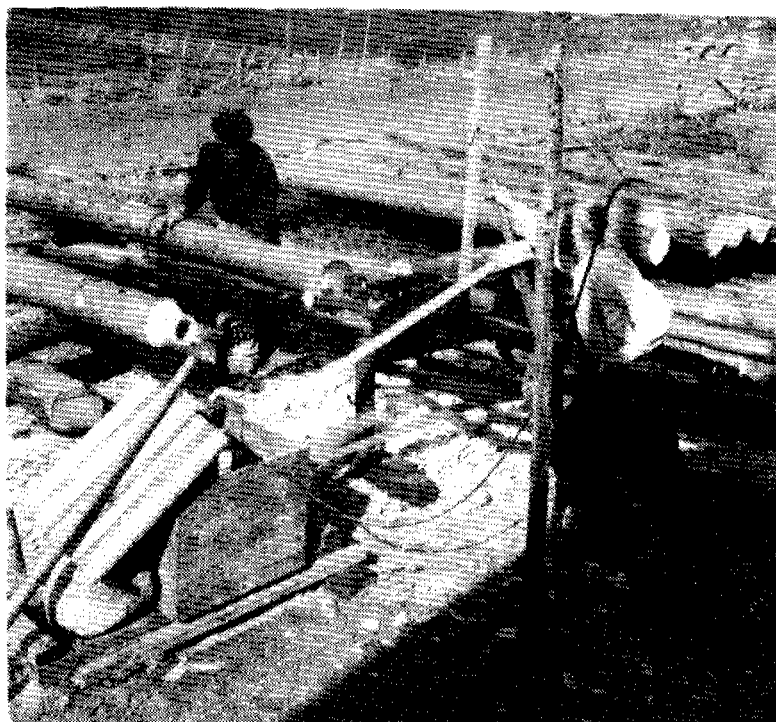
Fig. 22. Machine-boring of wooden pipes in Ilmajoki (Western part of Finland) in the late 1950's. (Photo: M. Viitasaari).
