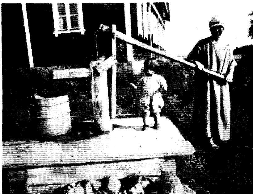
Fig. 12. Well equipped with a wooden handpump in Mouhijärvi (Western Finland) in 1933. (Photo: National Board of Antiquities).
