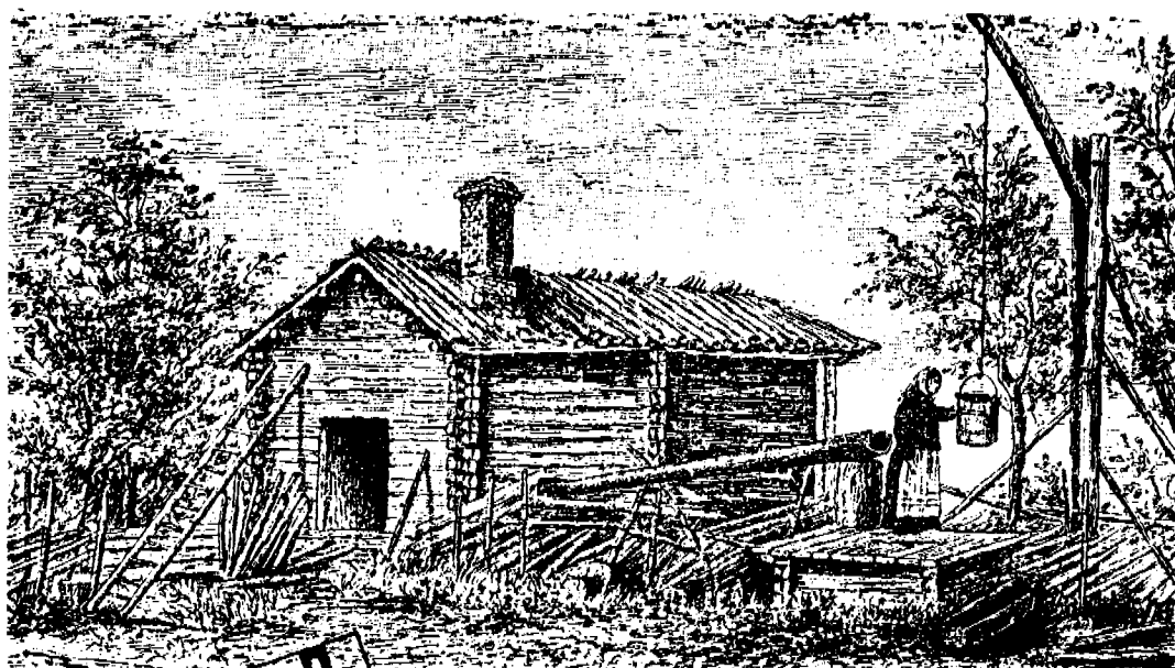
Fig. 7. Counterpoise lift well with a trough discharging to sauna in Janakkala (Southern Finland) in the 1880's. (Drawing: Heikel 1887).
