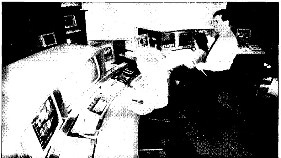
PLCs can be programmed to communicate information to the control room automatically.
