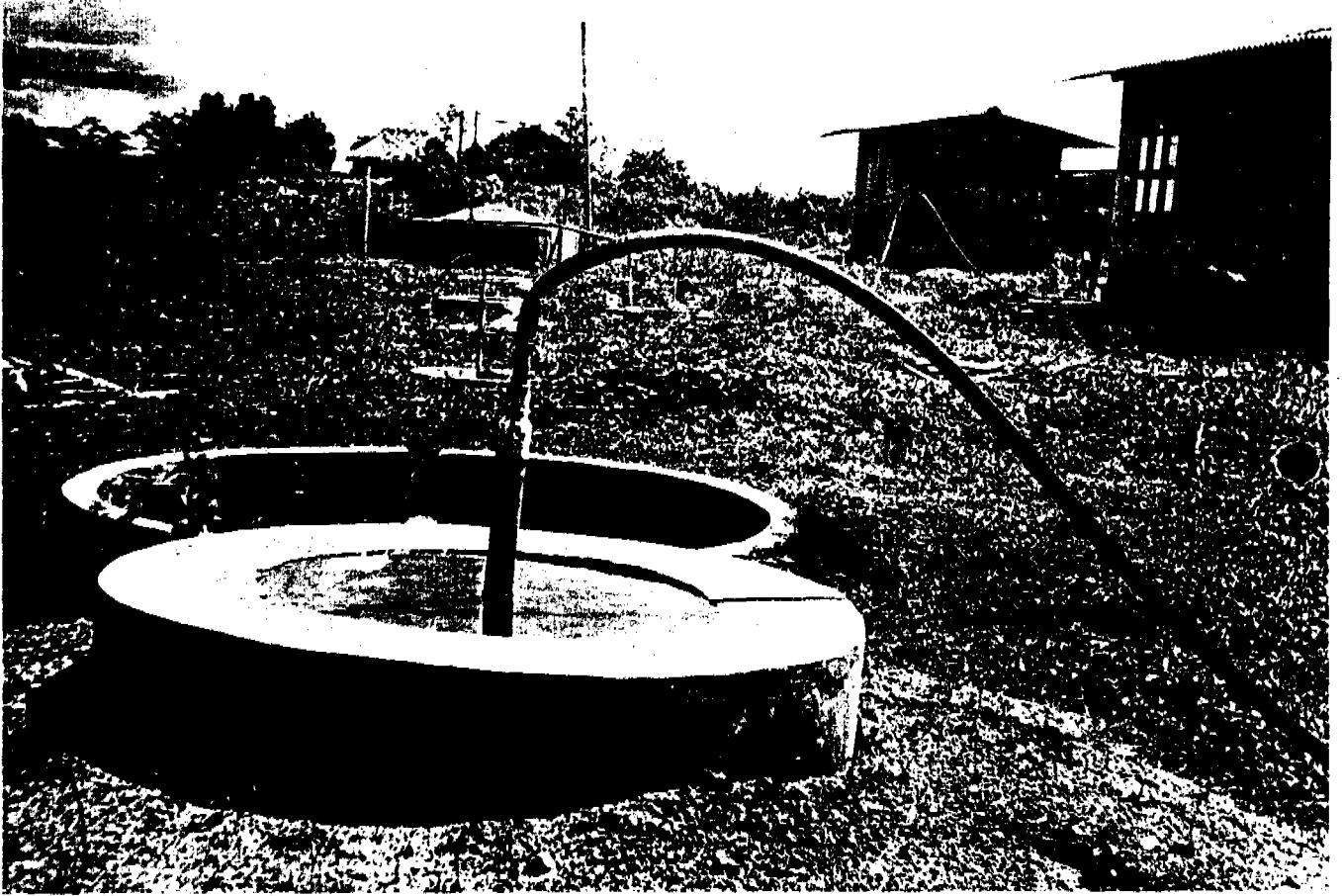
Biogas Unit -- Farm School, Angunu Kolapellessa
