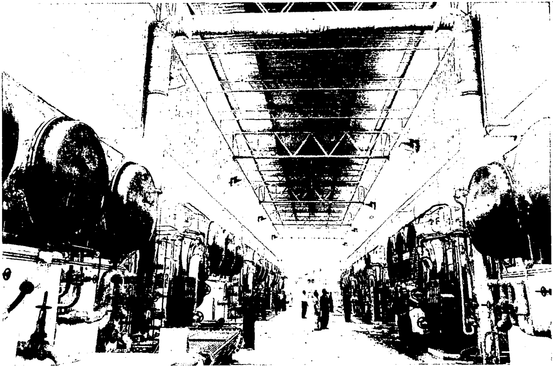
Figure 3. Shuwaikh 'A' Distillation Plant
