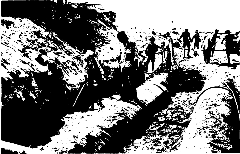
Figure 17. Installation of sanitary sewerage system in Abu-Dhabi. Pressure, gravity to 10 bars. Total length 90 km. Diam. 1200 – 1300 mm.
