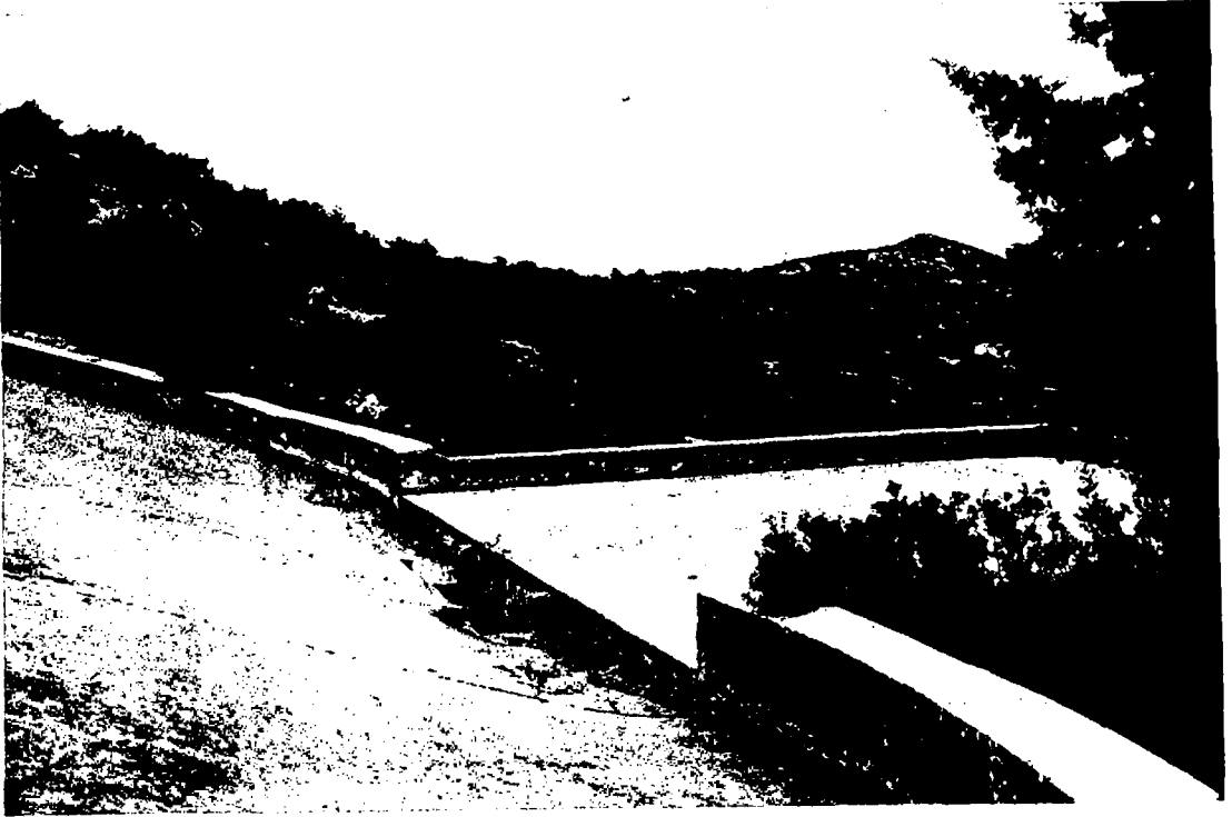
Fig. 2. Collecting surface and inlet of a cistern in Yugoslavia
