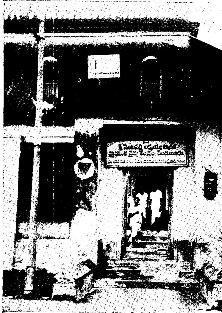
Primary Health Centre building at Tenduluru West Godavari Dist.
