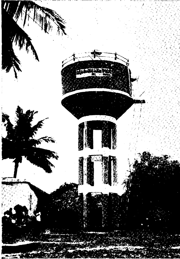
Over Head Service Reservoir.
