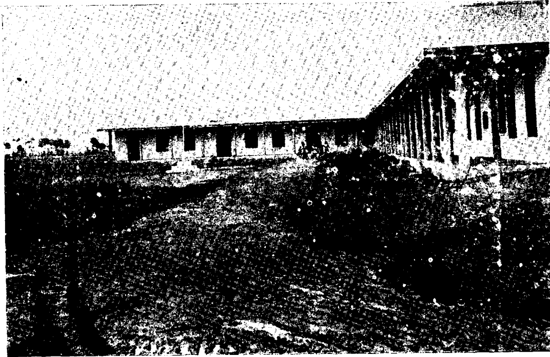
Another View of the High Schcol Building
