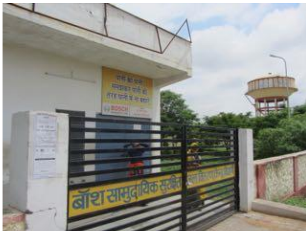
Figure 4-1 The Naandi plant in Vidhani (closed at the time of this visit at midday)
