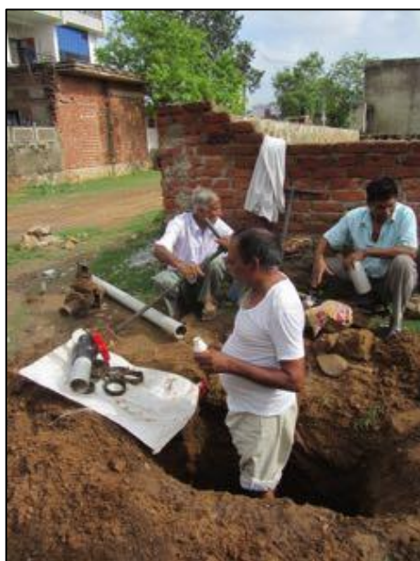
Figure 4-2 The pump operator at Boytawala replacing an old valve
