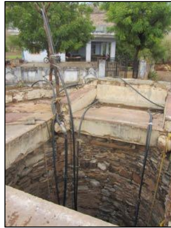
Figure 3-2 Community Johad built with the help of TBS, and an unprotected open well used by the same community for drinking water. Multiple households have installed individual electrical pumps to provide water.
