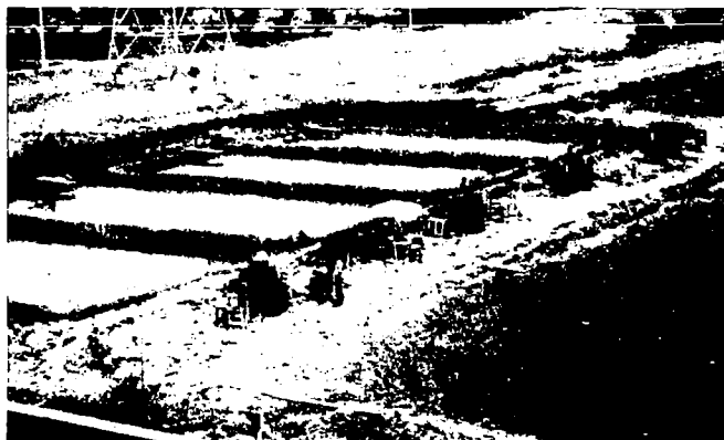
Fig. 4 Four 3.5 m 3 ferrocement digesters adjacent to four fish ponds (dimensions – 10 m wide, 20 m long and 1 m deep). The slurry from the digesters was collected and stored in a 1 m 3 storage tank to make a composite slurry sample prior to feeding.
