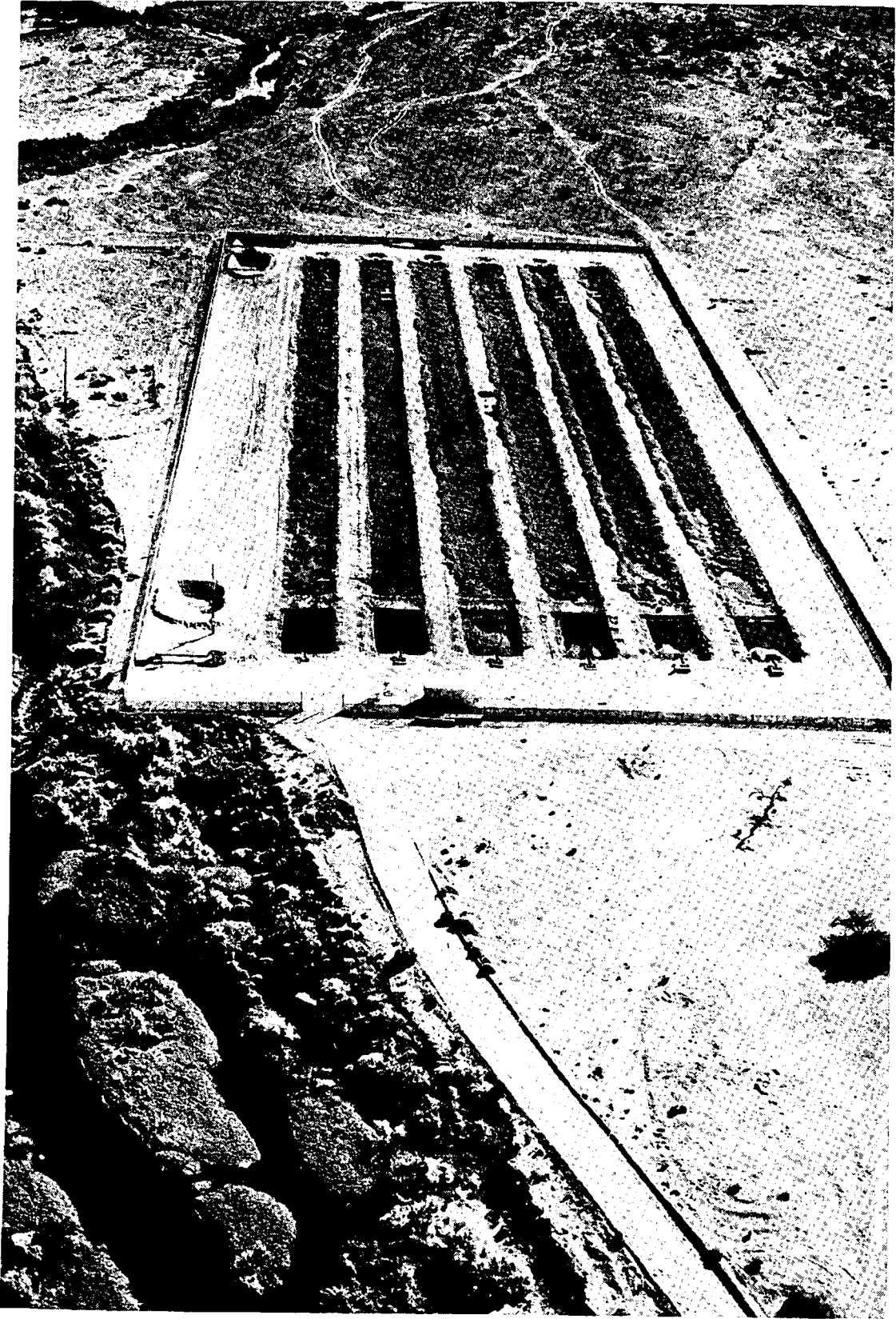
AERIAL VIEW OF FLUSHING MEADOWS PROJECT
