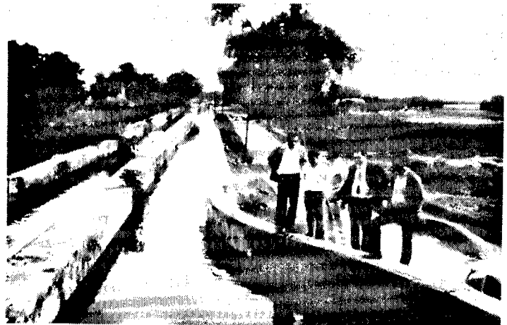
Photo 4.2 Outfall 1 of the Kanpur (U.P.) wastewater force main. The wastewater is used to ir- rigate 1300 ha of rice, wheat, forage and flower fields
