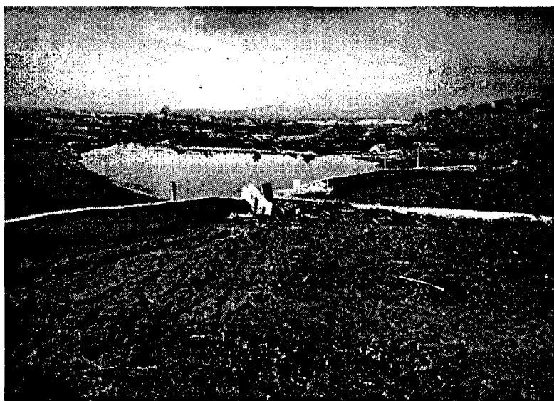
Scum Covered Settling Tank (foreground) and Anaerobic Ponds (background)
