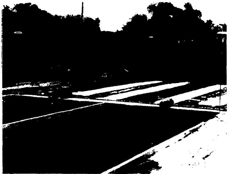
Figure 6-3.—Paved rectangular heated drying beds, Dunedin, Fla.
