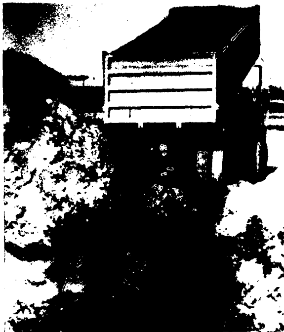
FIGURE 11-14 UNLOADING SLUDGE INTO WIDE TRENCHES WAUKEGAN, IL
