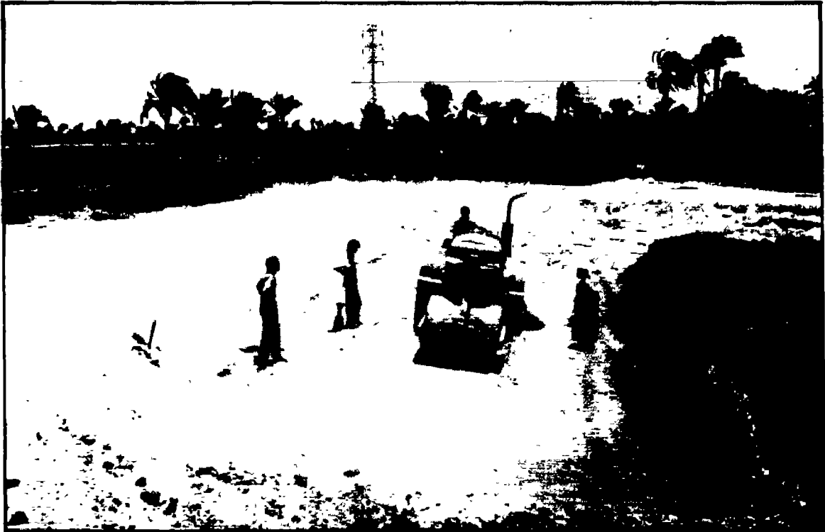
EMBANKMENTS EXECUTION IN WELL COMPACTED LAYERS
