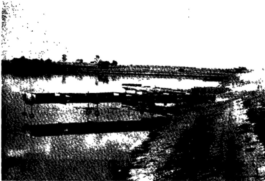
Fig. 7.17 Outlet structure on final maturation pond at the line A before it filled up after remedial work was done. Note the paving slabs are in place.
