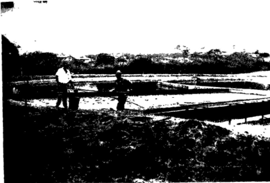
Fig. 7.5 workmen removing scum using dippers at Embu
