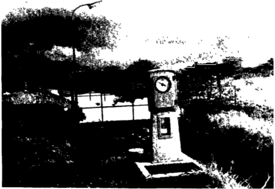
**Fig. 7.14** Gauge measuring effluent from final maturation pond on line B. Note the frothing that occurs
