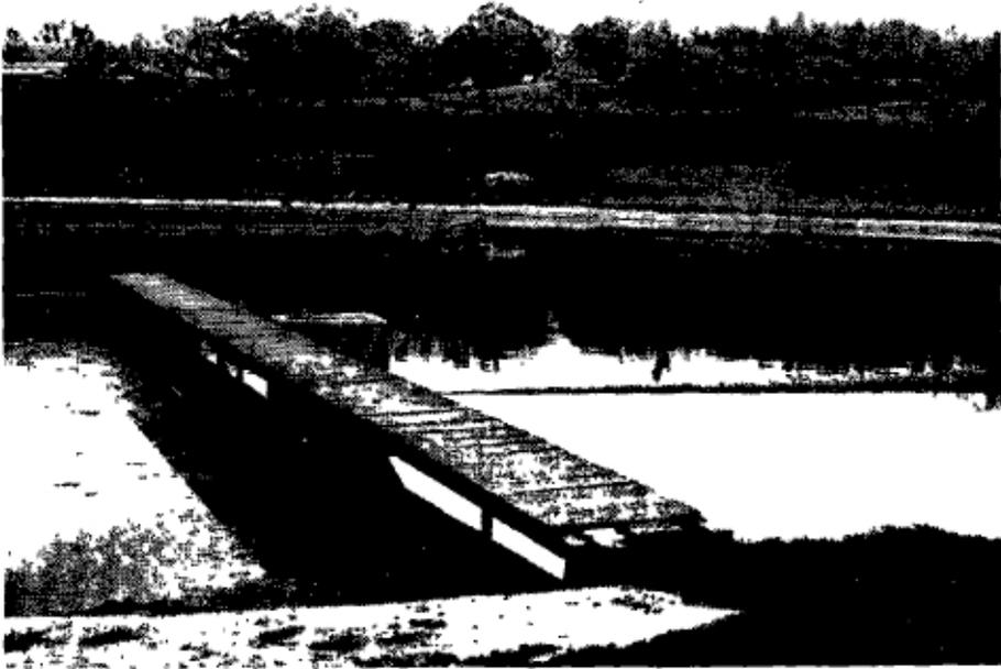
Fig. 7.4 shows submerged inlet pipe and scum baffle at Embu Primary pond
