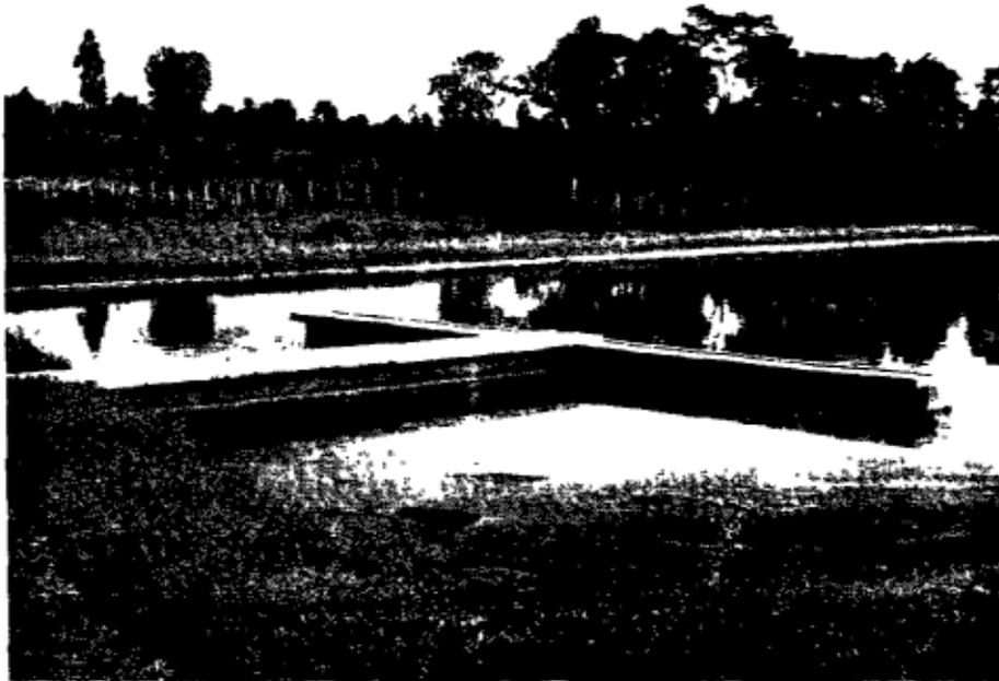
**Fig. 7.1 showing Karatima inlet to primary facultative pond - Note: the scum at bottom of picture**
