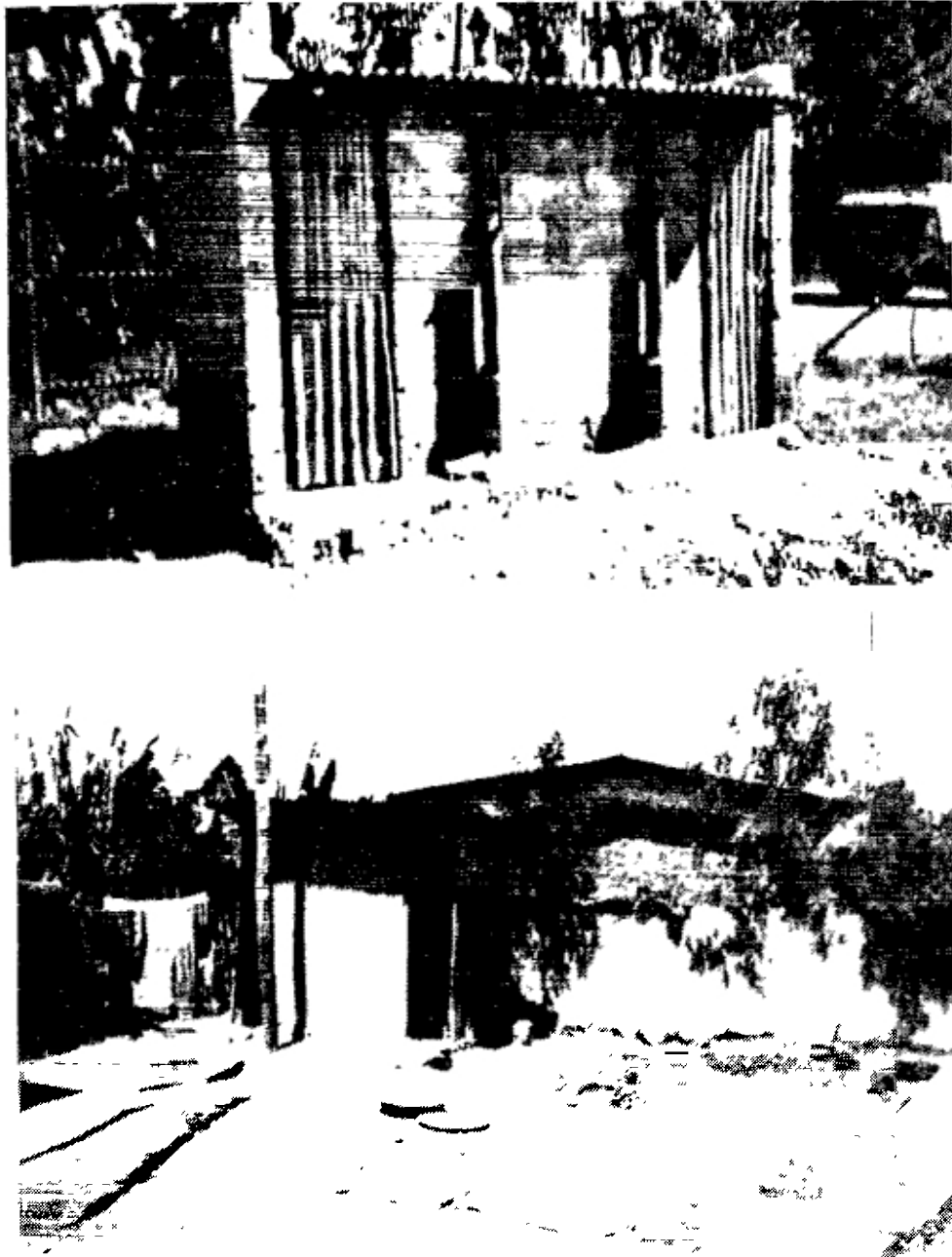
Figure 5. Typical ventilated and unventilated pit latrine in Addis Ababa.
