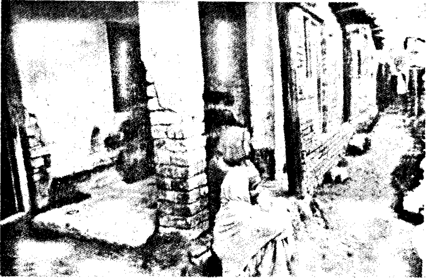
Sulabh Shauchalaya tanks in the verandah of a house.
