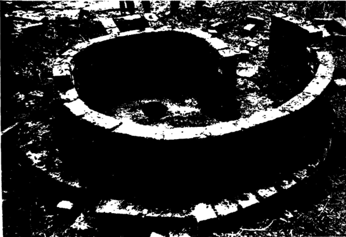
Figure H. Building up the superstructure and vent pipe
