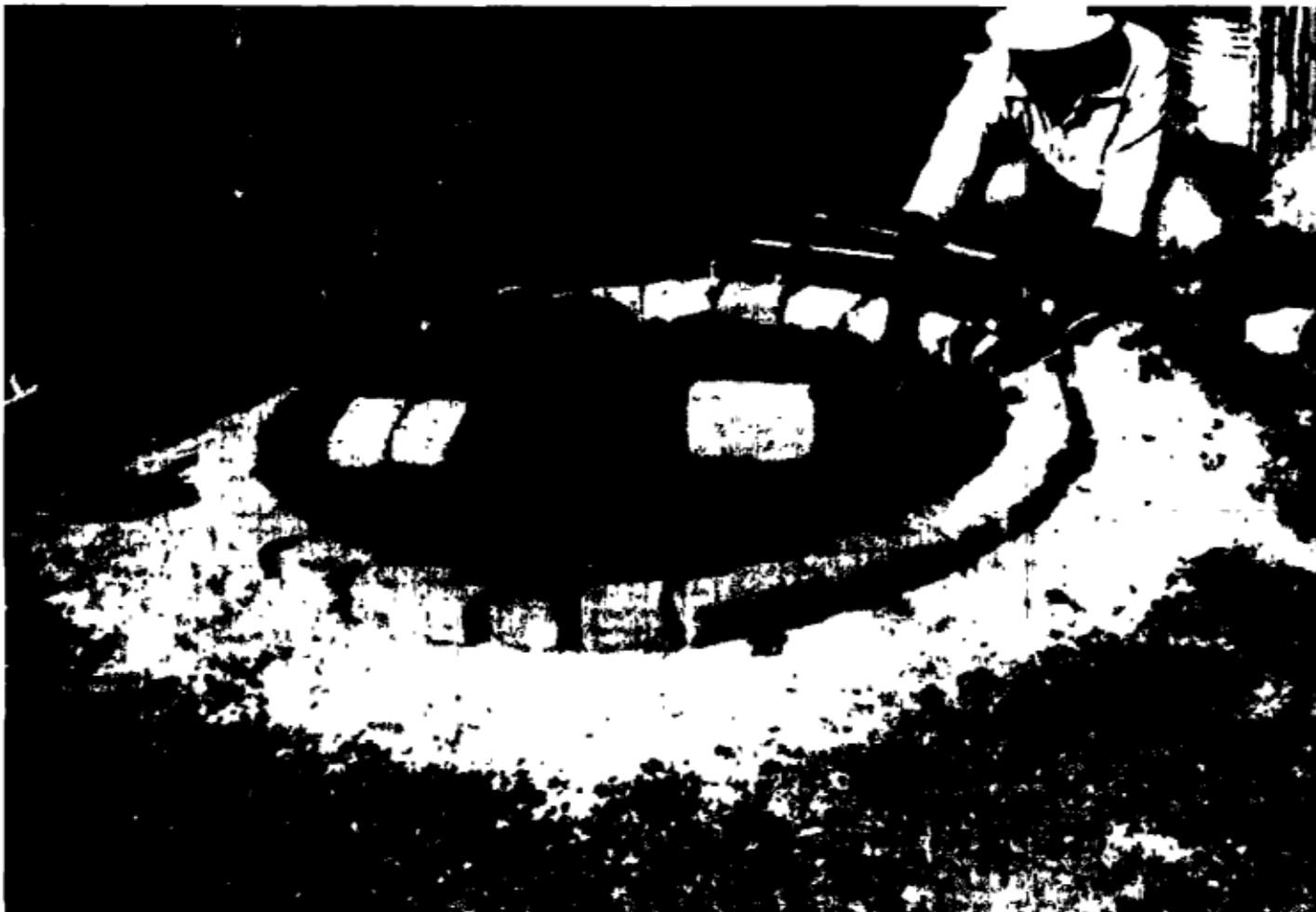
Figure E. Casting the reinforced concrete coverslab on site.
