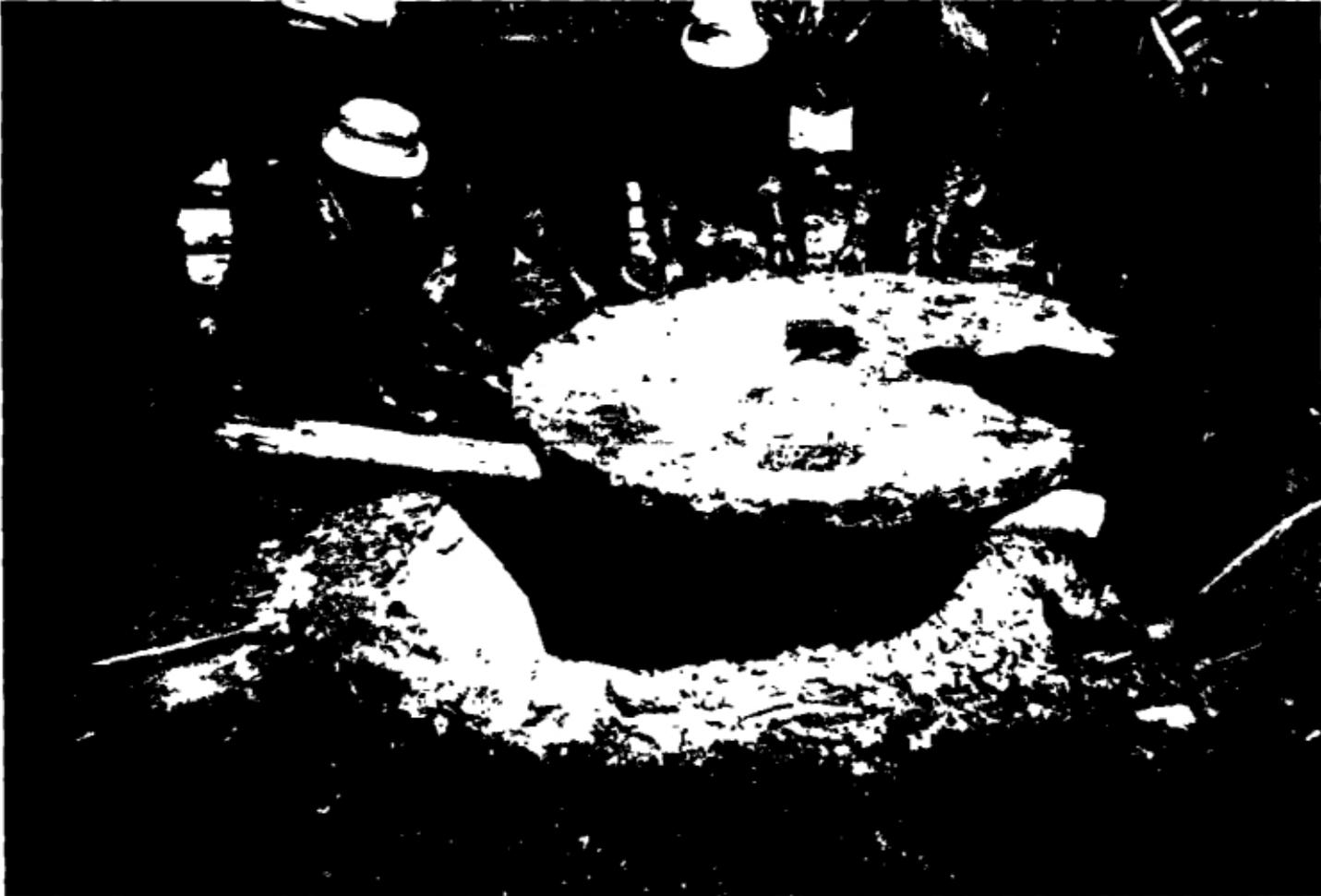
Figure F. Placing the coverslab on the brick collar.
