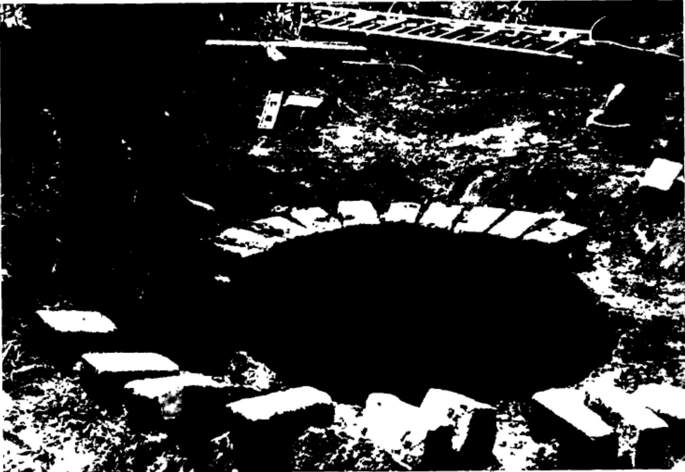
Figure D. Laying the brick collar.
