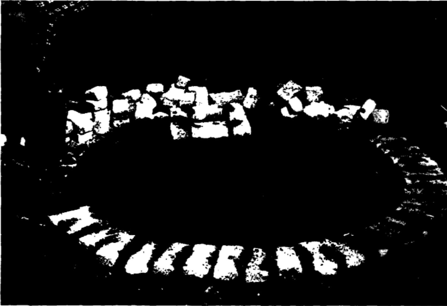
Figure G. Laying the brick foundation for a round spiral superstructure.
