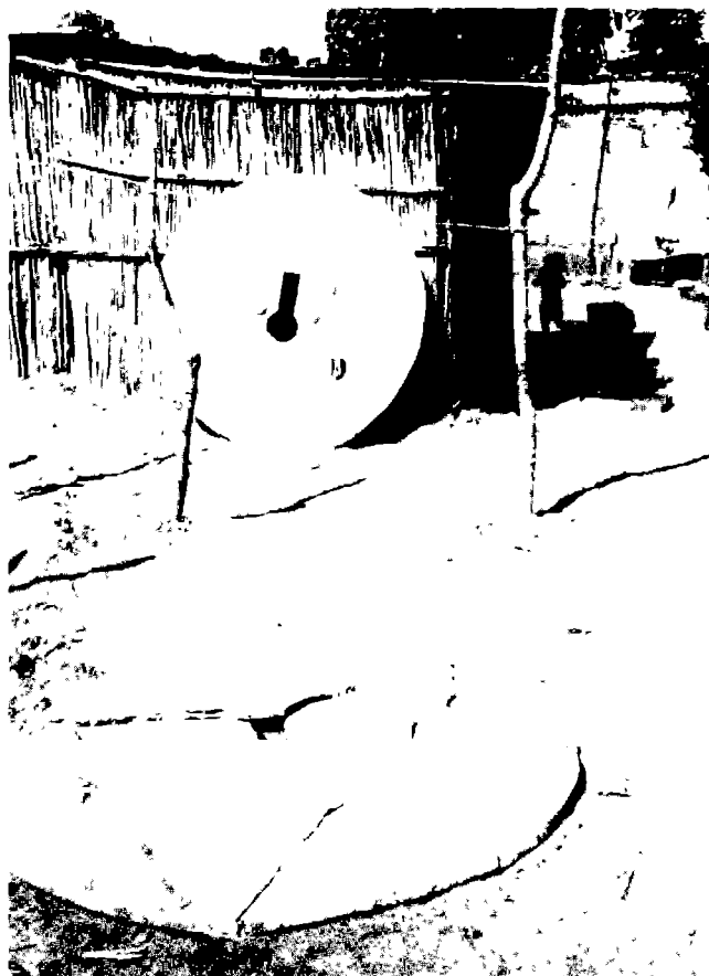
Fig. 8 Experiments were made with ventilated latrines. Here, a slab did not pass the security test.
