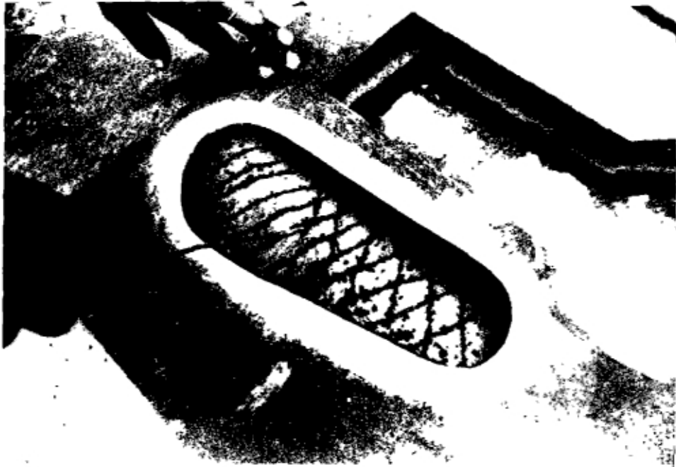
Fig. A-13 The surface is scratched to allow the cement to bond better.
