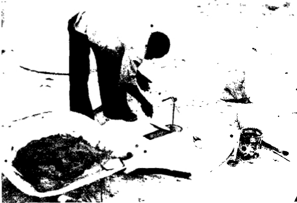
Fig. A-17 The lid is cast in the hole of the slab in which it is to be used. The iron is bent for the handle. The mason who made the slab also makes the lid and foot-rests. He then has a personal responsibility for the final product. As his initials are on the slab and the lid, any weaknesses in his work can be easily identified and corrected.
