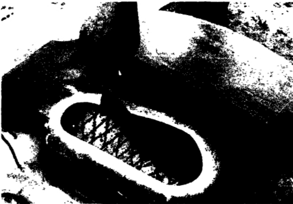
Fig. A-20 The foot-rests are made of stone-free cement mortar (1 part cement : 3 parts river sand). The mason starts by cleaning and wetting the scratched surface.
