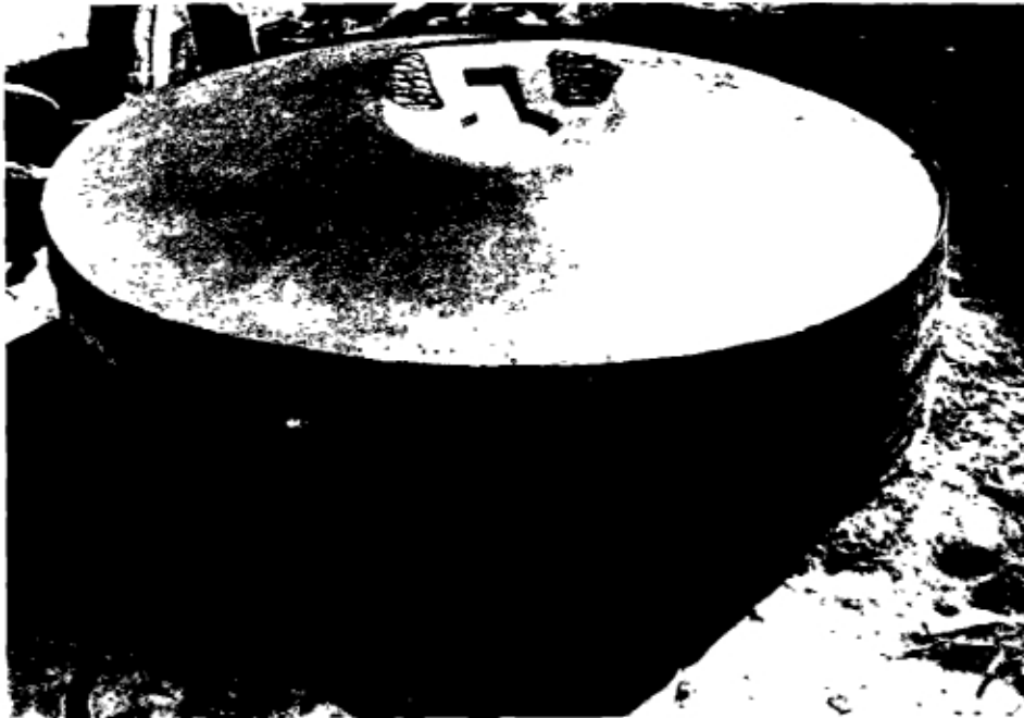
Fig. A-16 By raising the mould, several slabs can be made one on top of another, casting a new one each day. After 1 week, the pile is dismantled to make the lids and foot-rests.
