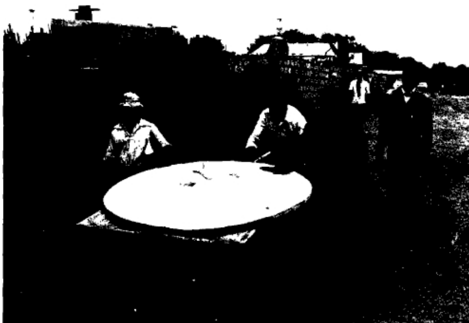
Fig. A-26 To transport the slab a two-wheeled cart is used. One man from the workshop accompanies the cart to ensure that it will be returned to the workshop.
