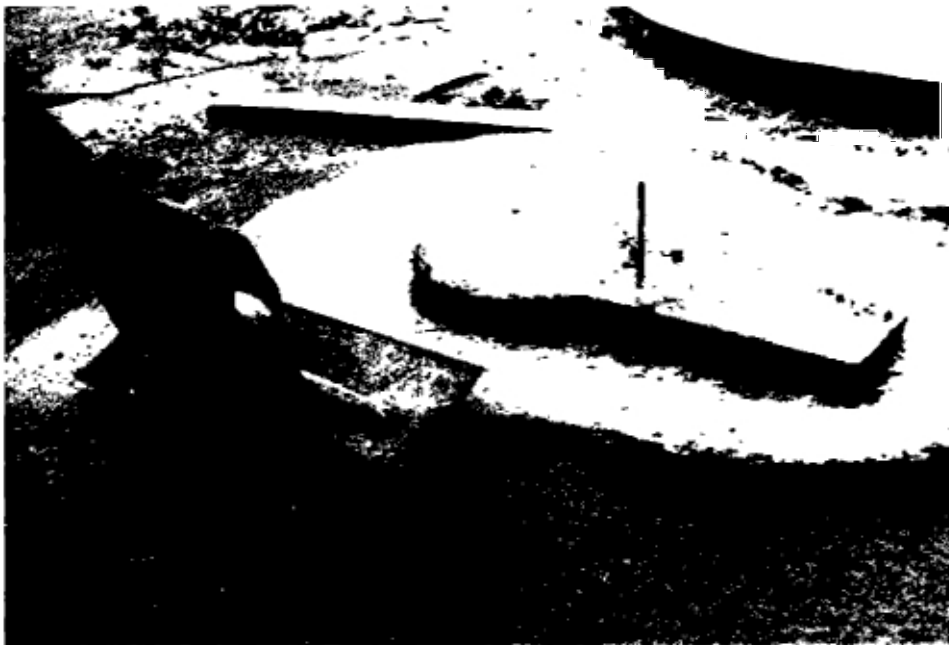
Fig. A-10 The surface of the slab is then smoothed out.
