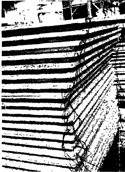
SEPTIC TANK SIDES. NOTE CONSTRUCTION TIE WIRES
