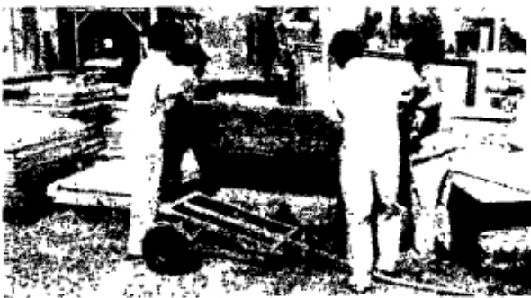
STACKING PANEL AFTER REMOVAL FROM MOLD
