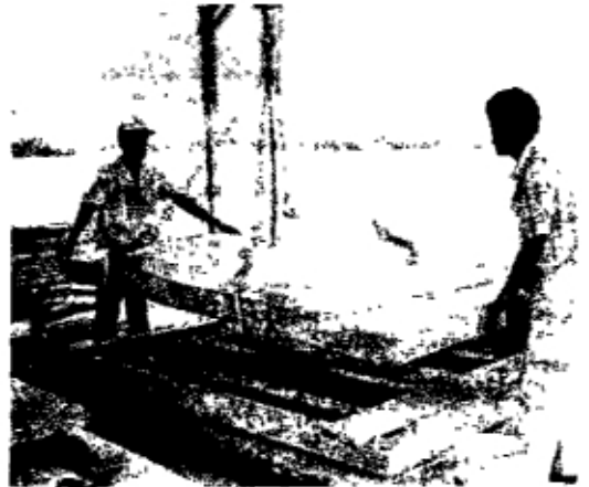
MOVING MOLD TO CURING STACK
