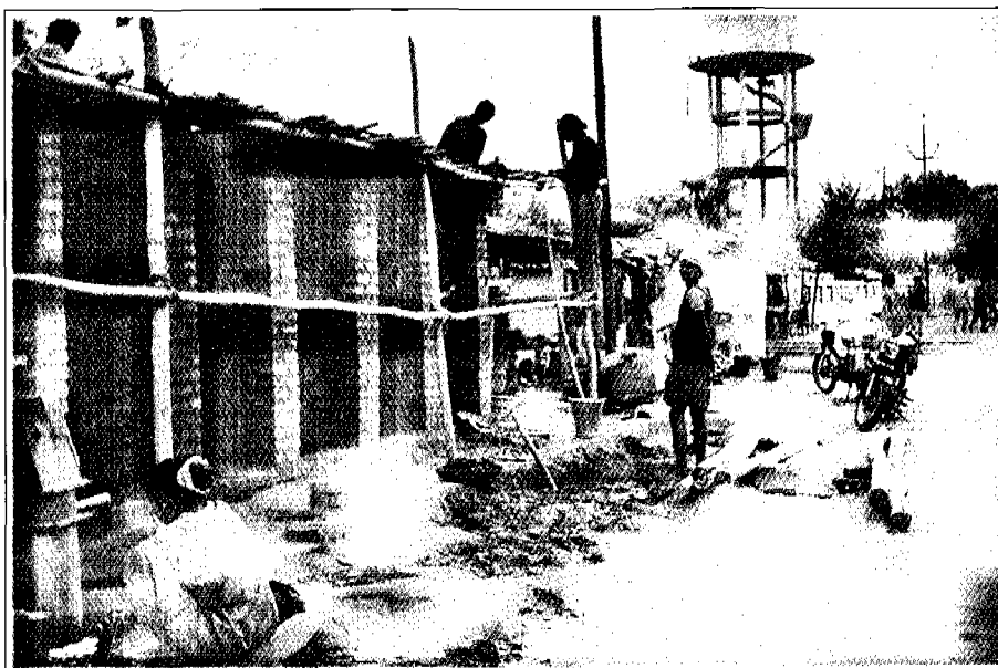
Community members constructing the toilet
