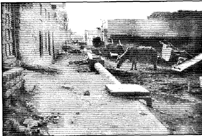
Figure 4.7 A community-built sewer in Faisalabad
