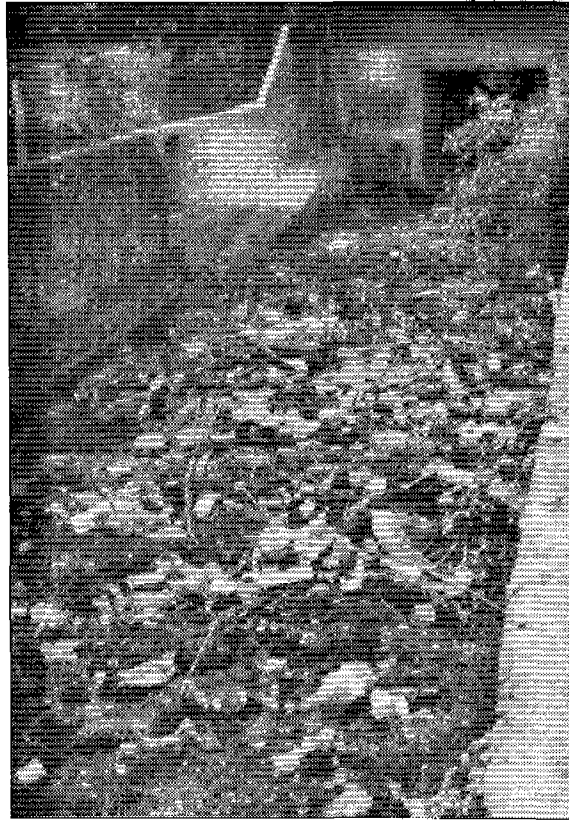
Figure 4.1 Sanitation problems are interconnected Solid waste blocking storm drain in Kathmandu, Nepal
