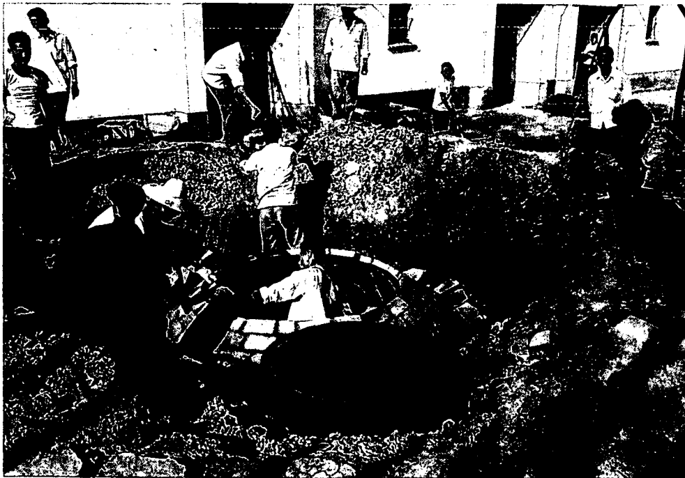
Fig. 24 Construction of a Chinese Biogas Plant
