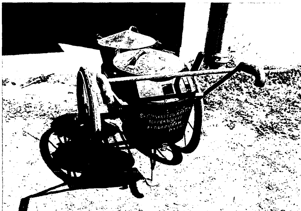
Figure 35 - Handcart with buckets for the removal of excreta
