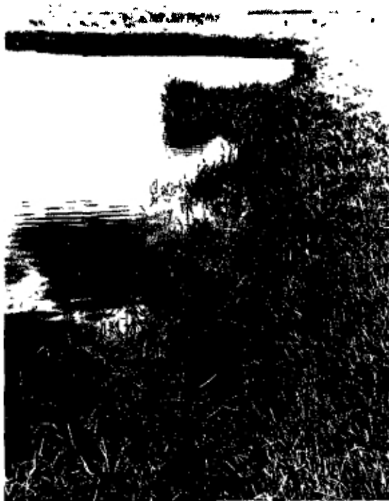
Plate 12 Two waste stabilization ponds. The banks of pond 1 are not properly constructed and extensive colonization of the pond by vegetation is taking place. This will reduce the pond volume and allow snail and mosquito breeding near the shore. The pond is unfenced and there is nothing to prevent the cattle from drinking from, or wading in, the pond. Pond 2 is well constructed and the banks are clearly being kept clean. A simple inlet arrangement is also shown. (Photos D. D. Mara)
