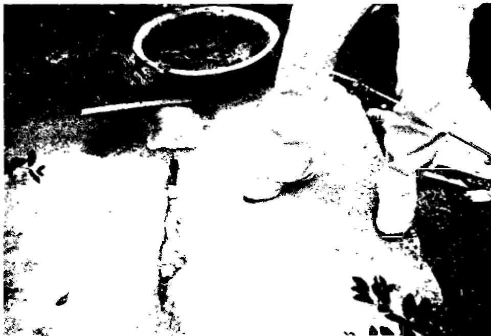
Plate 11 A crack like this in a septic tank cover can create an unbearable mosquito nuisance for the owner and his neighbours. After desludging, septic tanks should be carefully sealed, and preferably covered with earth (Photo S Cairncross)
