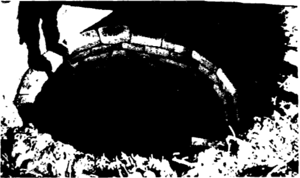
Plate 8 Open jointed brickwork lining in a round pit in Zimbabwe. A round pit is the most stable shape, so that no cement mortar is needed (Photo D D Mara)
